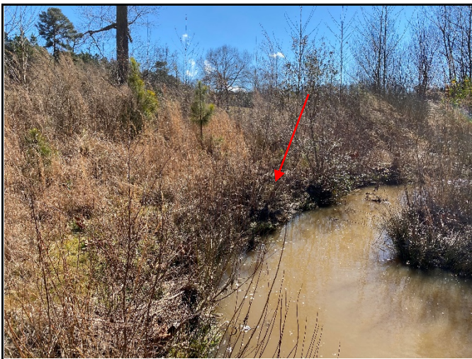
Previously repaired bend a long Reach R2 (photo: 2/16/21)
