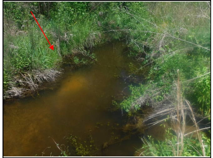
Previously repaired bend a long Reach R2 (photo: 5/5/21)
