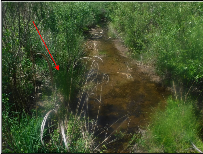
Previously repaired bend a long Reach R2 (photo: 5/5/21)
