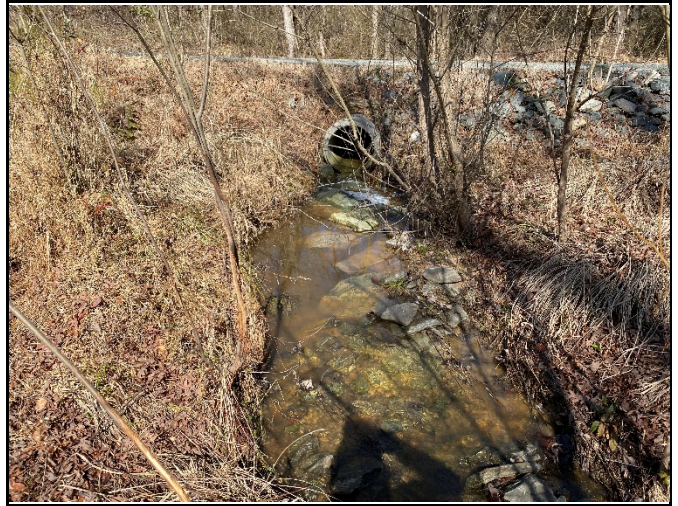
Flow in pipe culvert on R4 (photo: 2/16/21)
