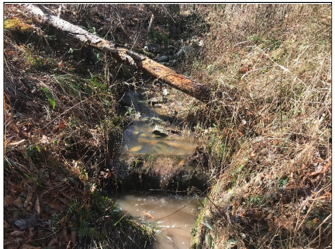
PP-42: Reach 7, view upstream at Station 10+40
