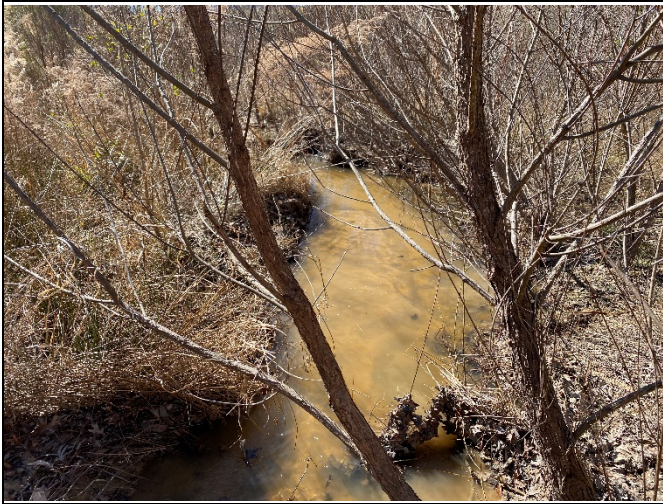
PP-25: Reach T1, view downstream at Station 11+75
