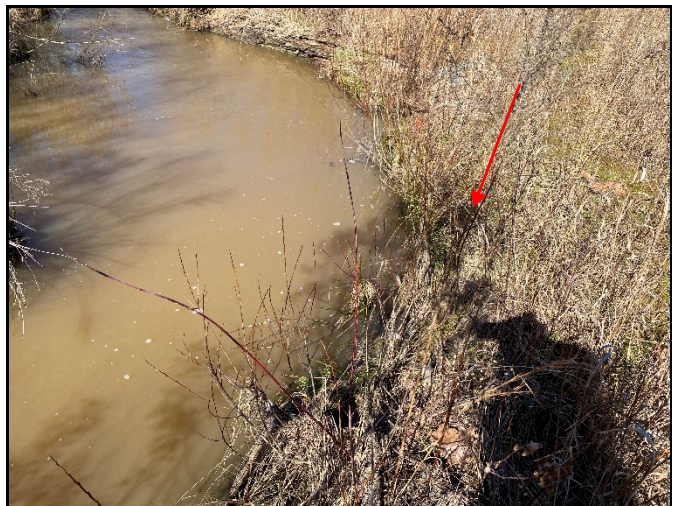
Previously repaired bend a long Reach R2 (photo: 2/16/21)
