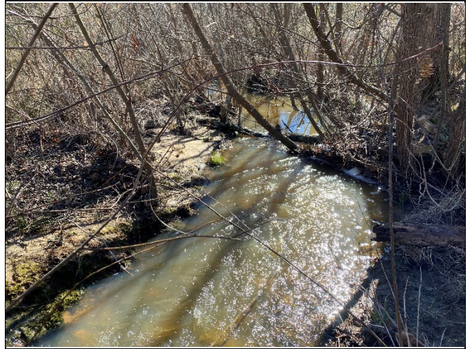
PP-32: Reach 2, view downstream at Station 39+40
