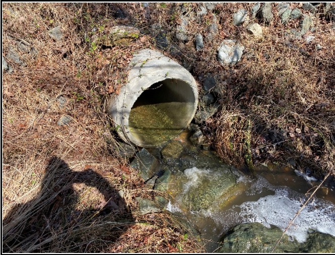
Flow in pipe culvert on R4 (photo: 2/16/21)
