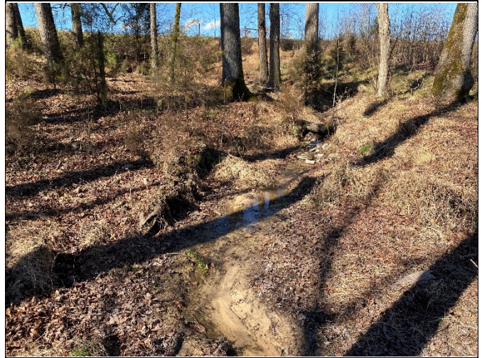
PP-58: Reach T2, view upstream at Station 10+80
