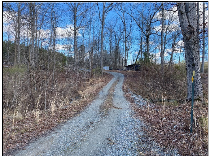
PP-6: Reach 3, stream crossing, Station 18+80
