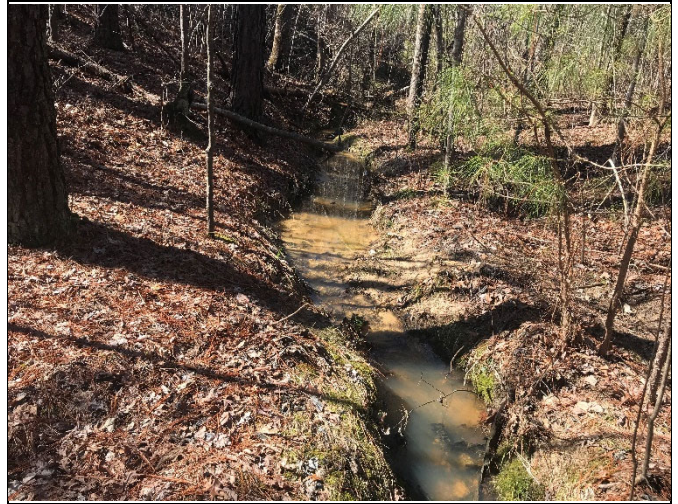
PP-44: Reach 7, view upstream at Station 15+00
