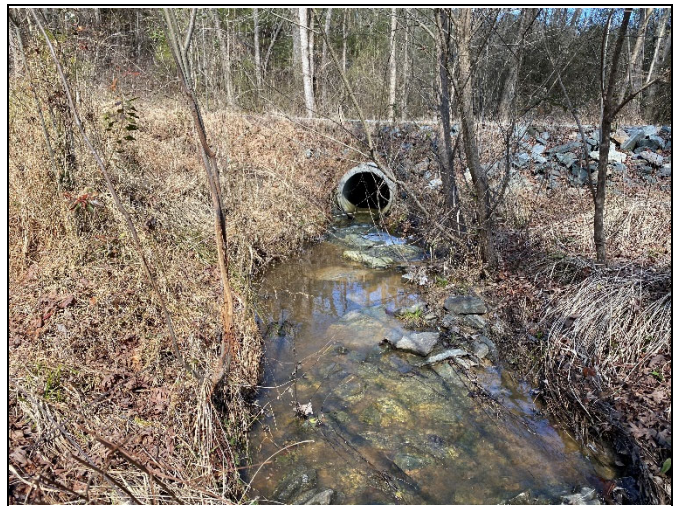
PP-12: Reach 4, view upstream at Station 10+50
