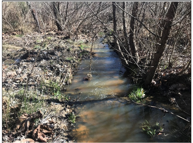
PP-48: Reach 5, view downstream at Station 32+50
