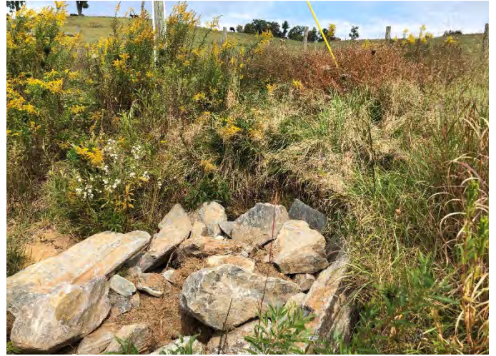
UT2 BMP – Headcut Repair 9-28-2021
