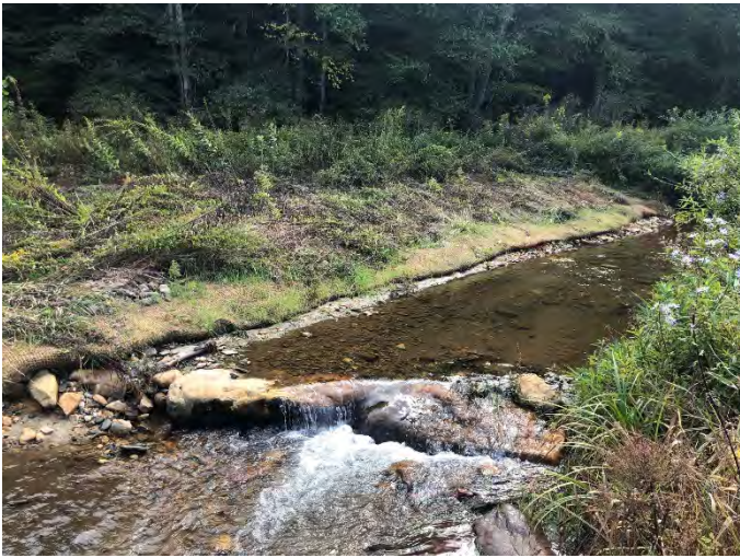
Vile Creek R2: STA 118+50 - 118+80 - Right Bank Repair 9-28-2021
