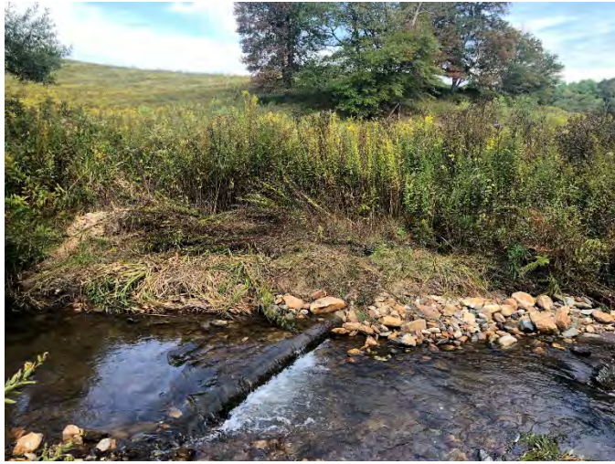
Vile Creek R2: STA 119+50 - 119+70 - Bank Repair 9-28-2021
