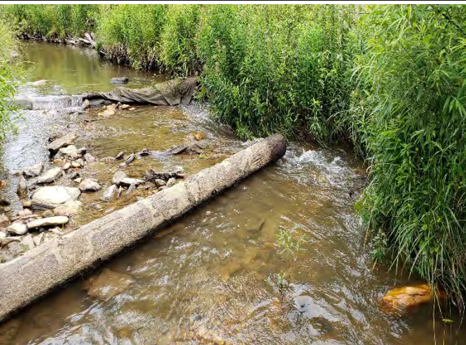
Vile Creek R2: STA 122+20 - 123+00 – Angled Log Riffle Failure. 7-01-2021
