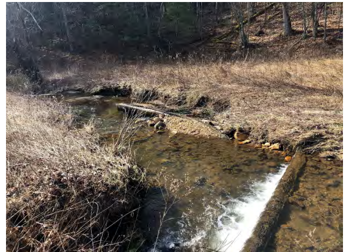
Vile Creek R2: STA 122+20 - 123+00 – Right Bank Erosion 3-17-2021
