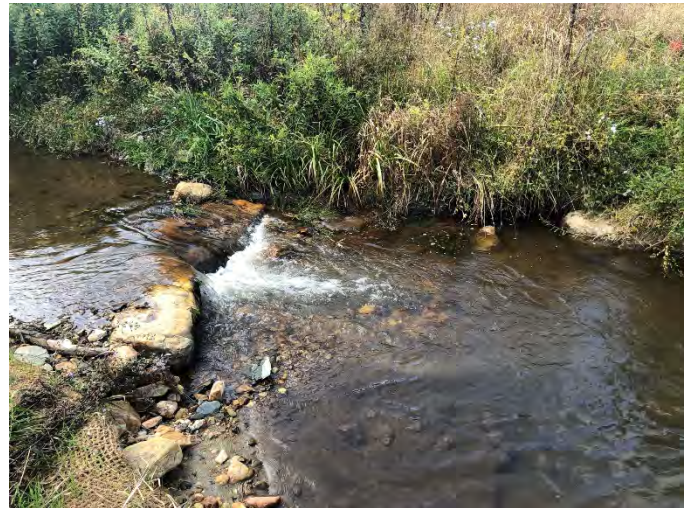
Vile Creek R2: STA 118+80 – J-Hook Repair 9-28-2021
