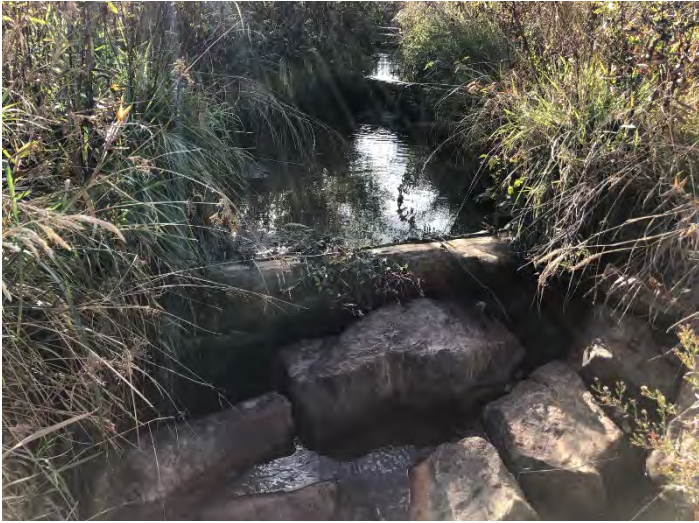
Photo 7 – UT1 R1: Station 212+50 – Structure piping. 10-26-2021
