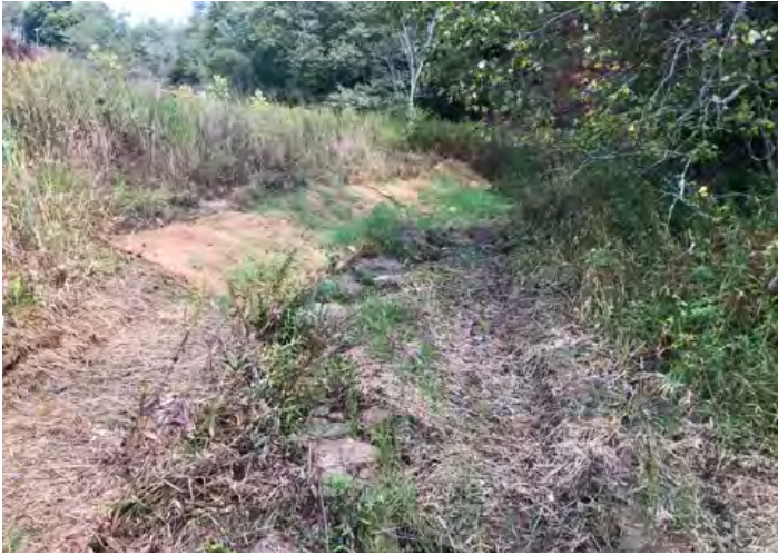
Vile Creek R3: STA 125+00 - 125+60 - Secondary Channel Repair 9-28-2021
