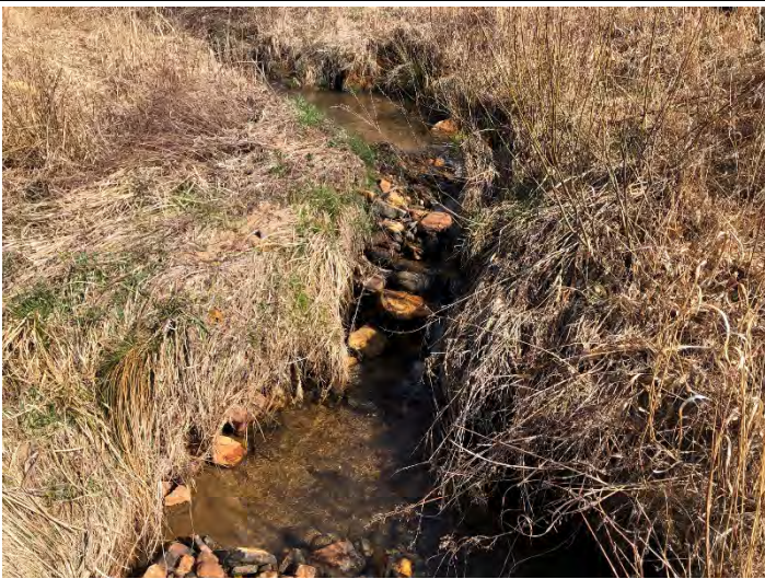
Photo 9 – UT2: Station 304+90– Headcut 3-17-2021
