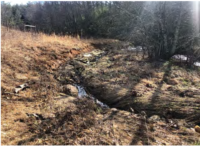
Vile Creek R3: STA 125+00 - 125+60 - Secondary Channel Erosion 3-17-2021
