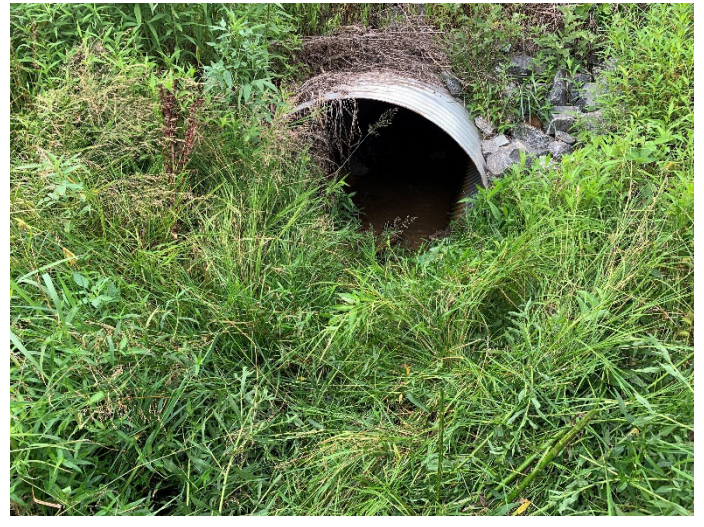
PP6A – view downstream—UT1 Reach 1B (06/29/2021)
