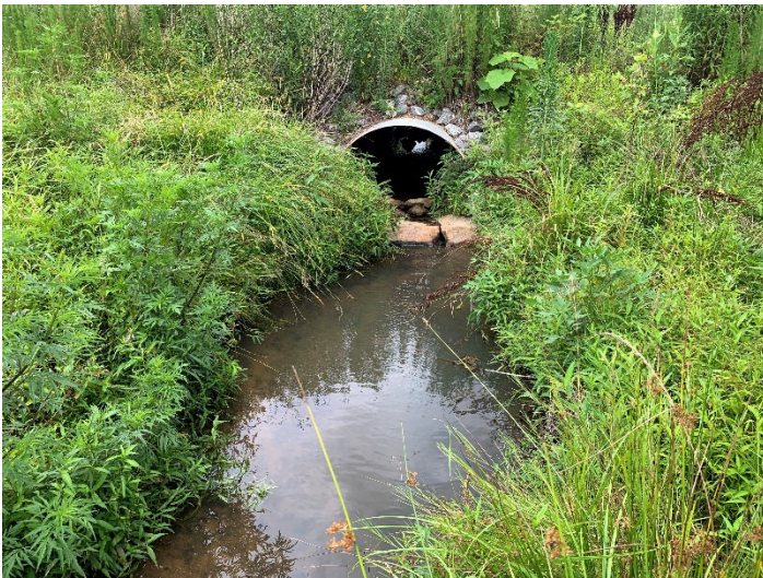
PP6B- view upstream—UT1 Reach 2 (06/29/2021)
