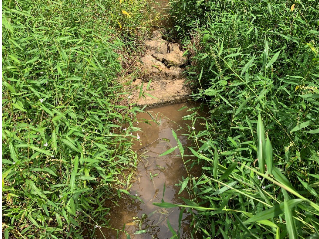
UT1 R1A Structure Piping (STA 104+00) – view Upstream (09/15/2021)
