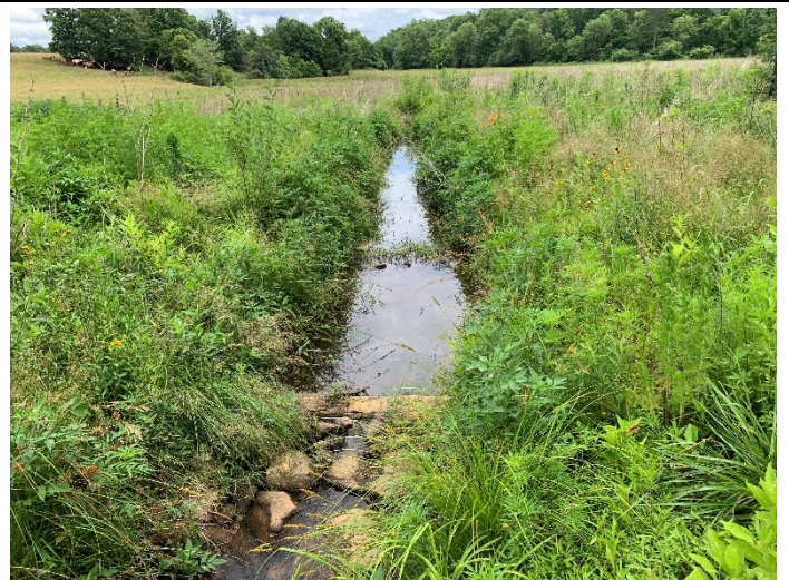
PP17 – view downstream— UT1 Reach 4B (06/29/2021)
