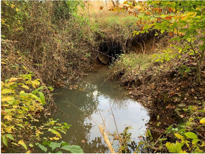
PP9B – view upstream—UT1 Reach 3 (11/03/2021)
