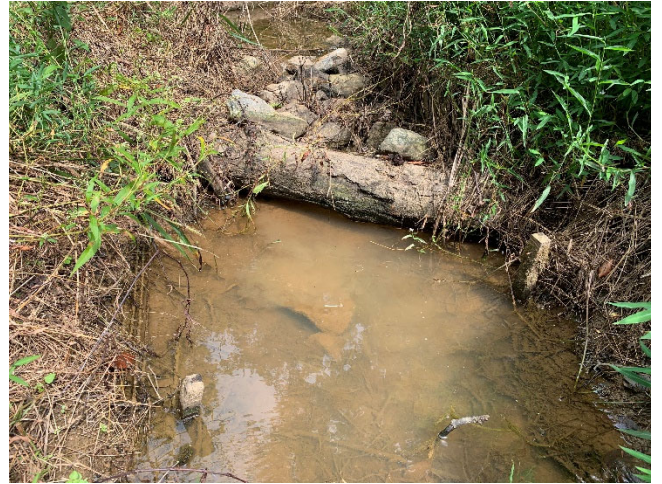
UT1 R1A Structure Piping (STA 104+00) – view Upstream (09/15/2021)
