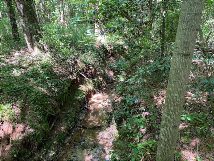
UBHC R1 Photo Point 1 – view upstream (6/17/2021)
