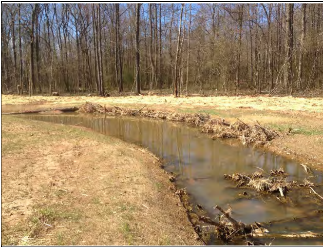
Hurricane Creek R1, As-Built (2015)
