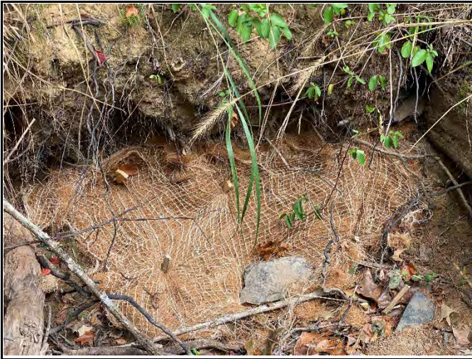
UT4-R2, SPA #1 Bank Repair (Right bank stabilized with matting, Close-up, Sept.2021)
