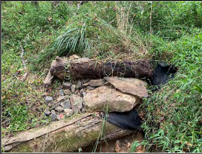
UT4-R1b, SPA #3 Bank Repair (scour filled-in with soil, matting and rock/logs installed on top, Sept. 2021)
