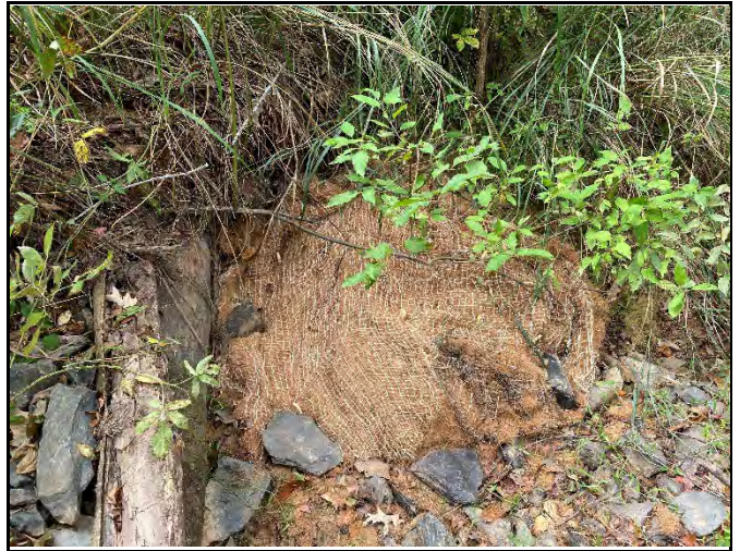
UT4-R2, Additional Bank Repair near SPA #1 (Stabilized with matting, Sept.2021)
