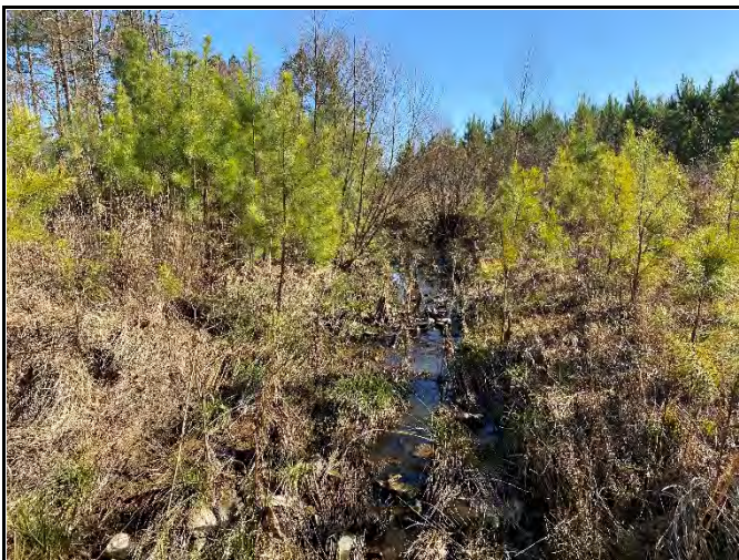
PP-17: Reach UT4-R4b – View upstream, Station 28+00
