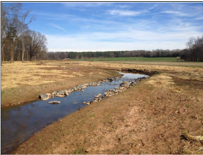
Hurricane Creek R1, As-Built (2015)
