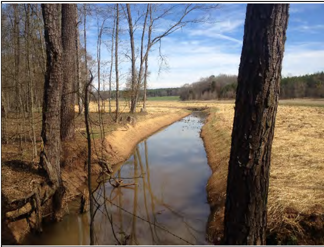
Hurricane Creek R1, As-Built (2015)
