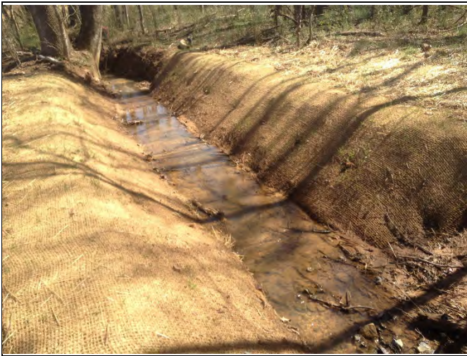
Hurricane Creek R3, As-Built (2015)
