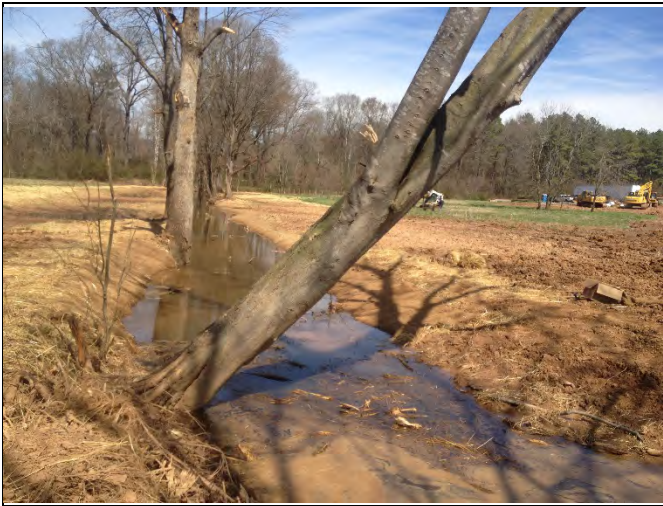
Hurricane Creek R2, As-Built (2015)
