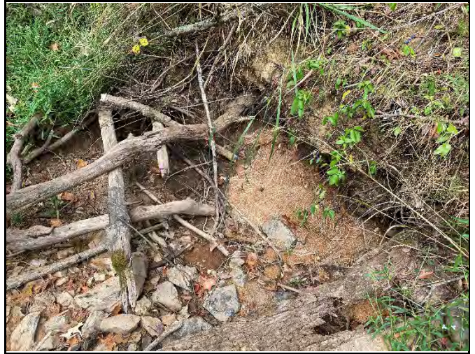
UT4-R2, SPA #1 Bank Repair (Right bank stabilized with matting, Sept.2021)
