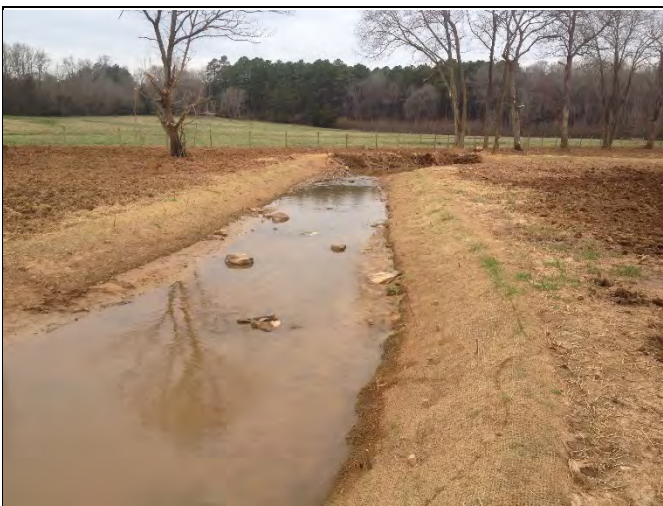
Hurricane Creek R2, As-Built (2015)
