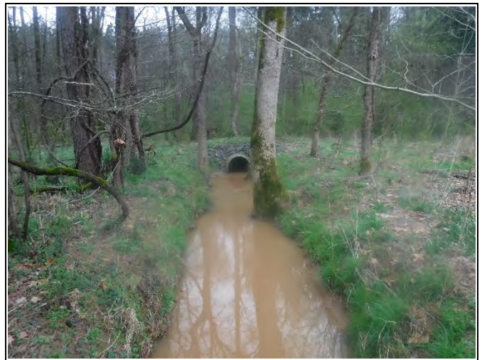
Hurricane Creek R3, MY7 (2021)
