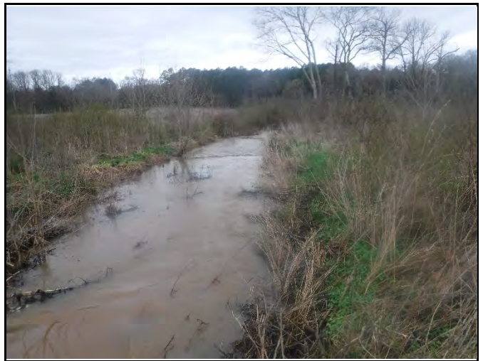
PP-16: HC Reach 2, view downstream at Station 36+00
