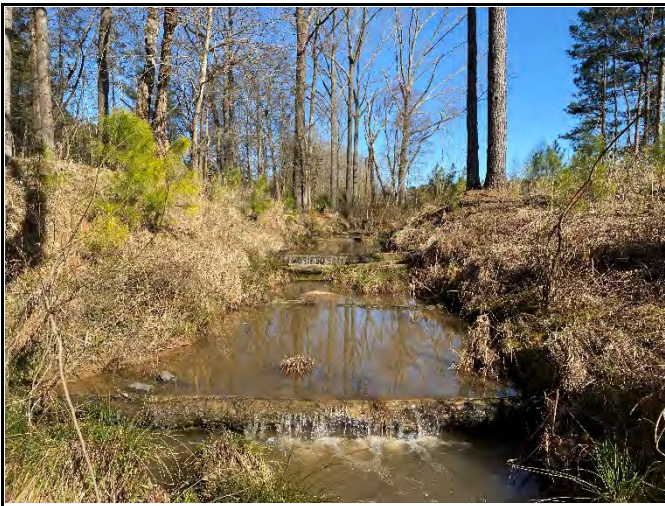
PP-23: Reach UT4-R2 – View upstream at Station 37+50
