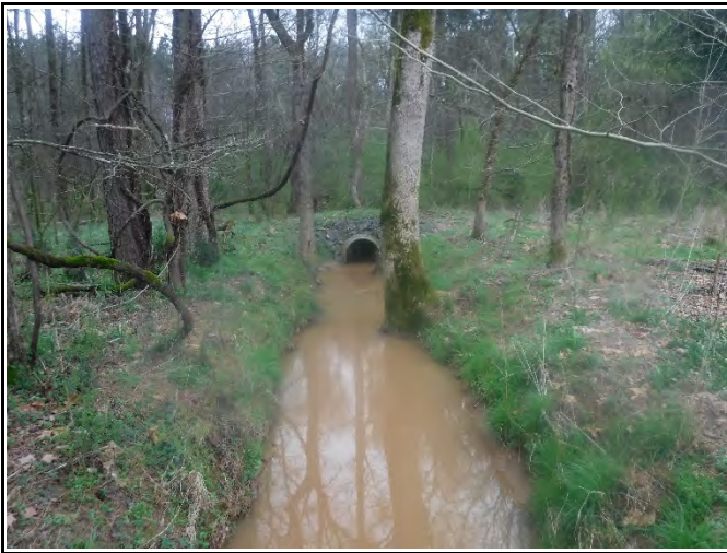
PP-21: HC Reach 3, view upstream at Station 11+40
