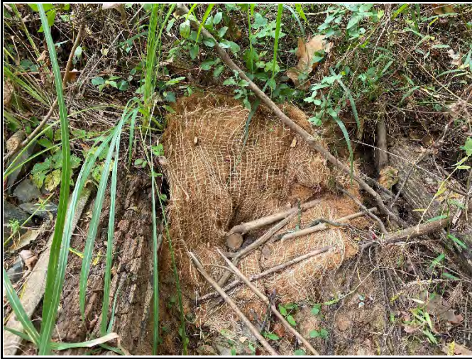
UT4-R2, SPA #1 Bank Repair (Left bank stabilized with matting, Sept.2021)
