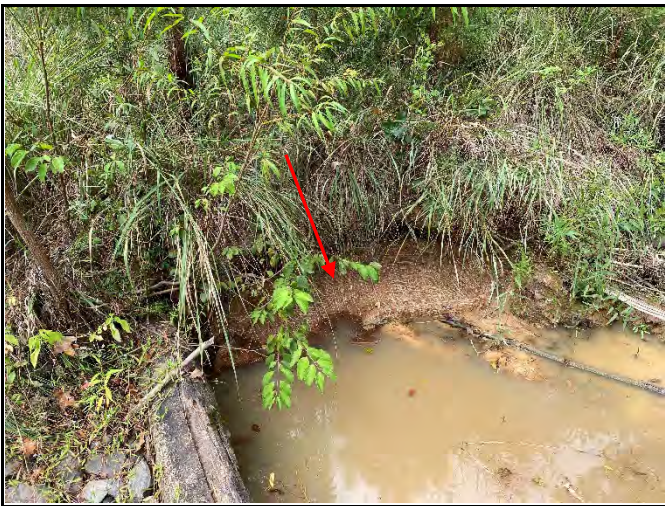
UT4-R2, SPA #2 Bank Repair (Stabilized with matting, Sept.2021)
