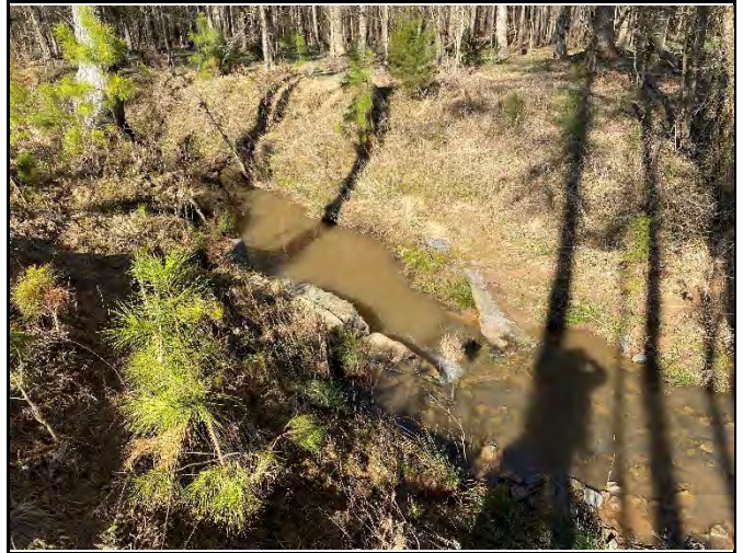
PP-20: Reach UT4-R3 – View downstream, Station 29+50
