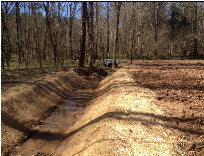
Hurricane Creek R3, As-Built (2015)
