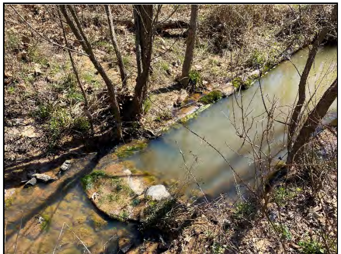
PP-54: Reach UT4-R 1b – View downstream, Station 13+25
