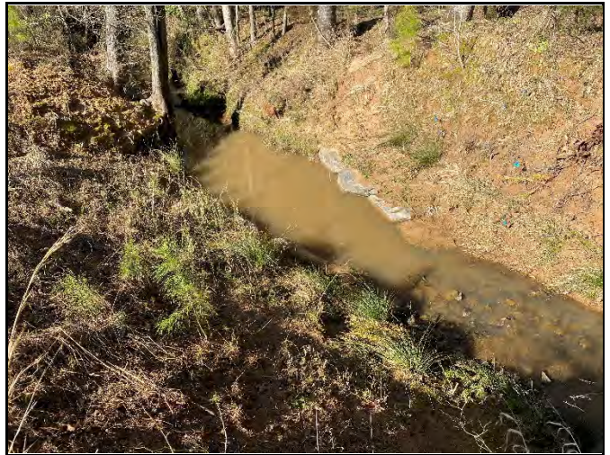
PP-22: Reach UT4-R3 – View downstream, Station 31+00
