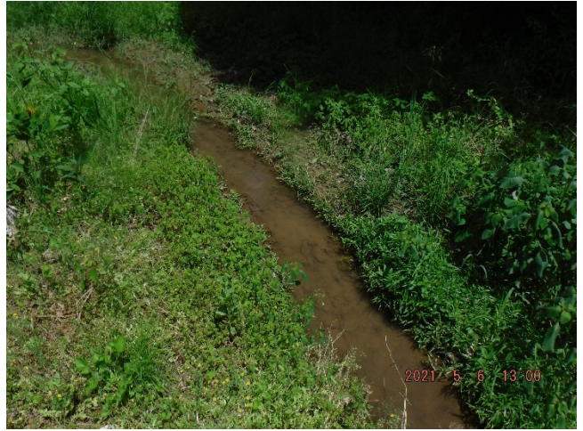
Candy Creek Reach 1 - Improved stream aggradation (Sta. 100+20-101+50) (5/6/2021)
