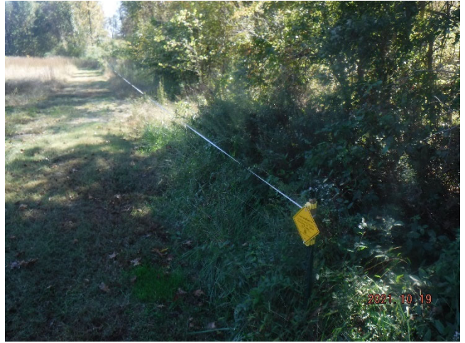
Candy Creek Reach 1 - Easement encroachment, RB (Sta. 111+00-113+00) (10/19/2021)
