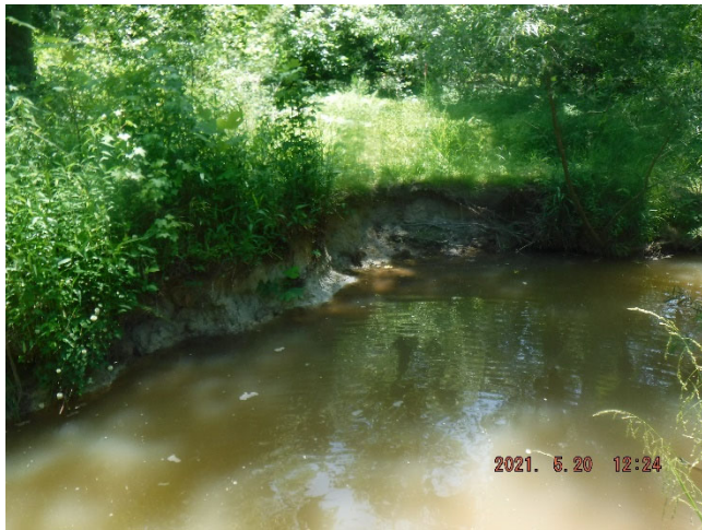
Candy Creek Reach 3 - Bank erosion, RB (Sta. 151+70-152+00) (05/20/2021)
