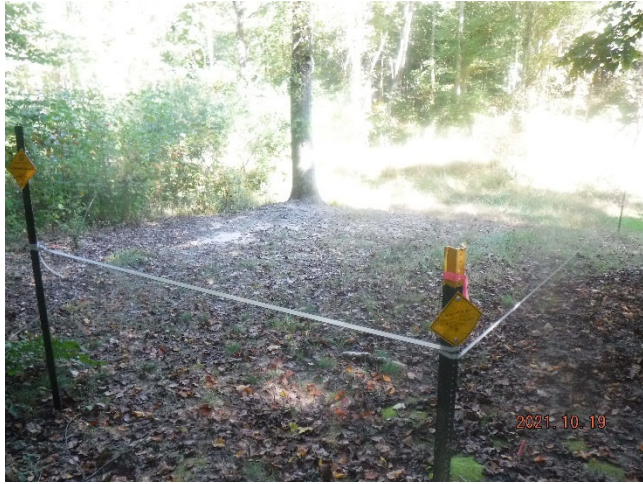
Candy Creek Reach 1 - Easement encroachment at upstream extent, LB (Sta. 100+00-100+60) (10/19/2021)
