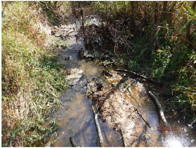
Candy Creek R2 - stream aggradation (Sta. 140+50-140+65) (10/07/2020)
