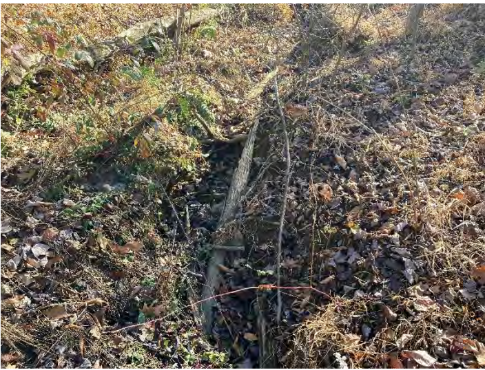
PHOTO POINT 8 UT2 R1 Headcut – upstream (12/7/2021)
