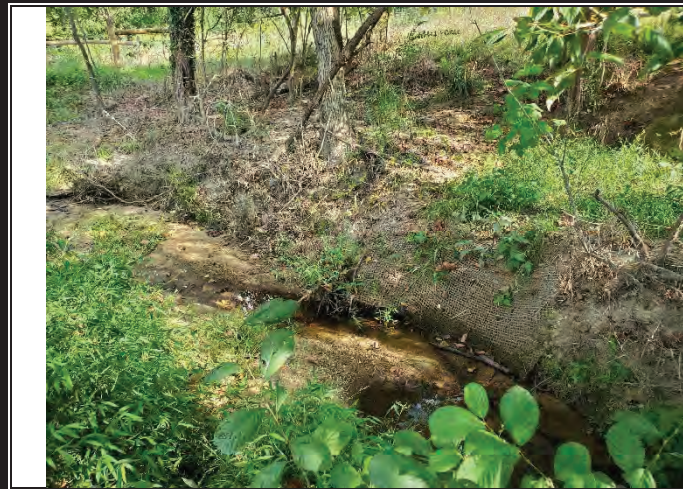
Figure 5.15 Stabilized section downstream UT MC (9/7/2021)
