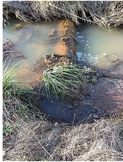
Wyant UT2 R3 – Structure Issue 322+00 (1/5/2022)
