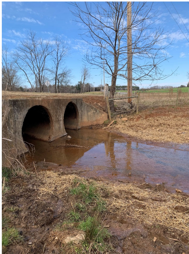
Wyant Road Culvert – Erosion mitigation through spreading of straw and seed (1/25/2022)
