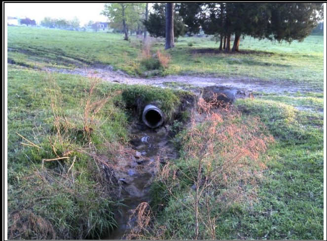
Existing downstream crossing along UT 2
