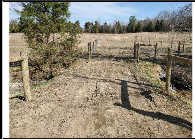
Figure 4.14 Installed Crossing Over UT MC (3/12/2021)
