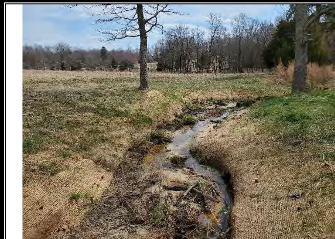
Figure 4.11 Stabilized Bank Along UT 2 (3/12/2021)
