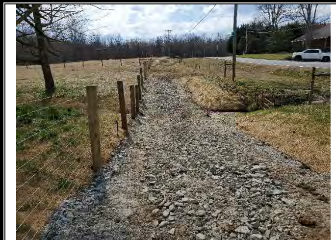
Figure 4.12 Installed Ford Crossing at Upstream Extents of UT 1 (3/12/2021)
