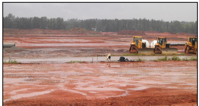
Example of extensive clearing and exposed soil which can result in very high erosion rates. Photo Credit: Rich McLaughlin.
