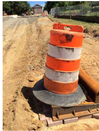
Pavement resurfacing on campus-owned road
