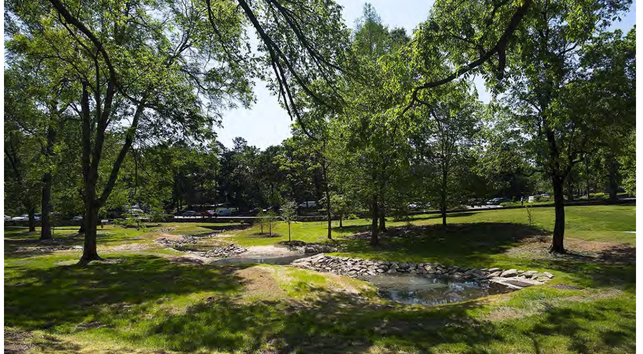
Battle Grove Regenerative Stormwater Conveyance
