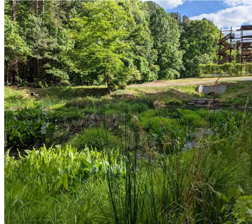
OEC Stormwater Wetland
