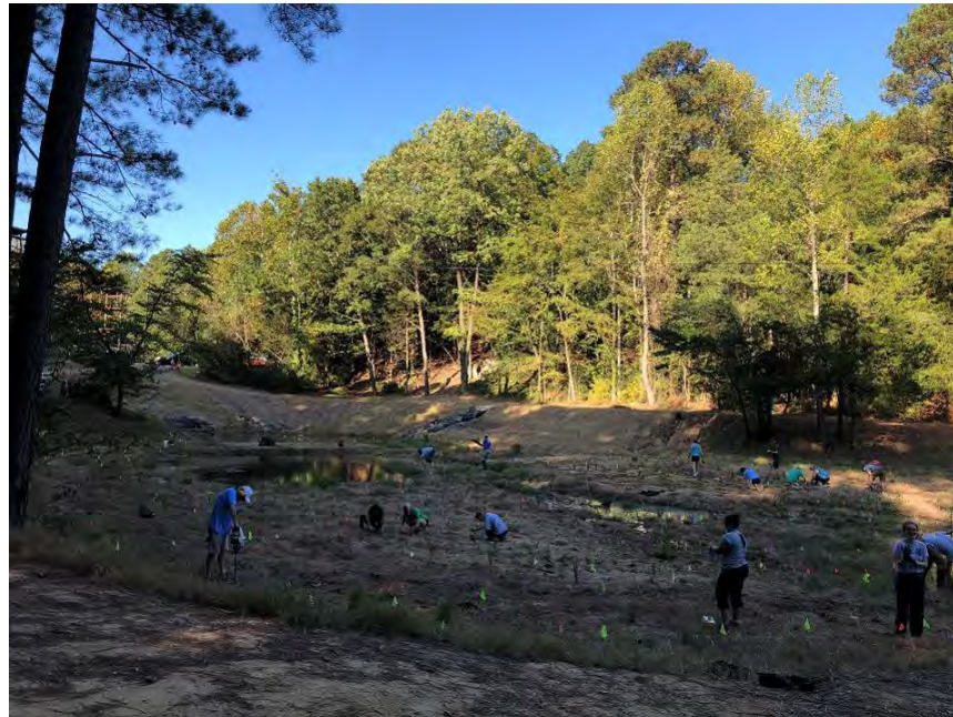
UNC staff planting stormwater wetland at Outdoor Education Center, 2020
