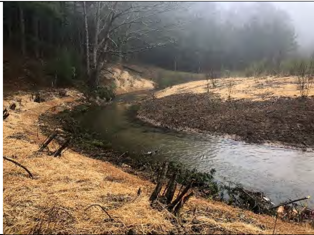
Brush toe geolift repair, left bank looking downstream
