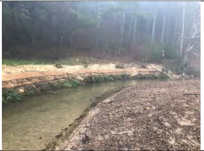
Brush toe geolift repair area from right bank, looking downstream
