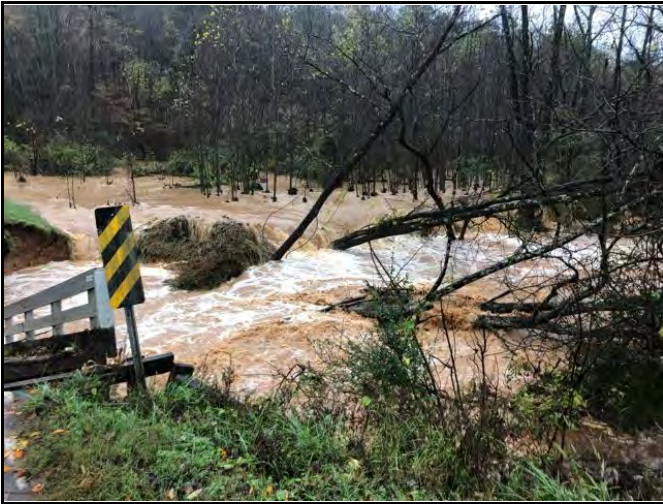
Flooding from Zeta remnants above the bridge upstream of R7 (10/29/20)
