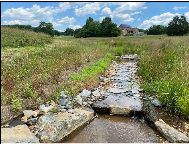
PP-41: Reach UT5, upstream, Station 15+00
