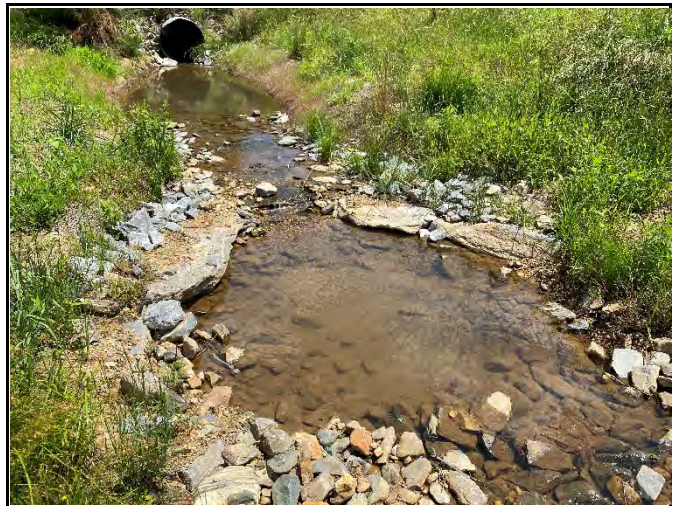
PP-48: Reach UT5, upstream, Station 10+50
