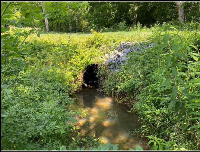
PP-37: Reach UT4A, upstream, Station 10+25
