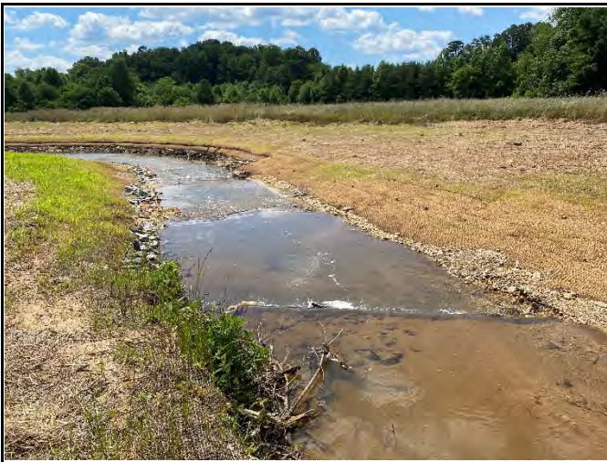
PP-11: Reach 7, downstream, Station 17+50
