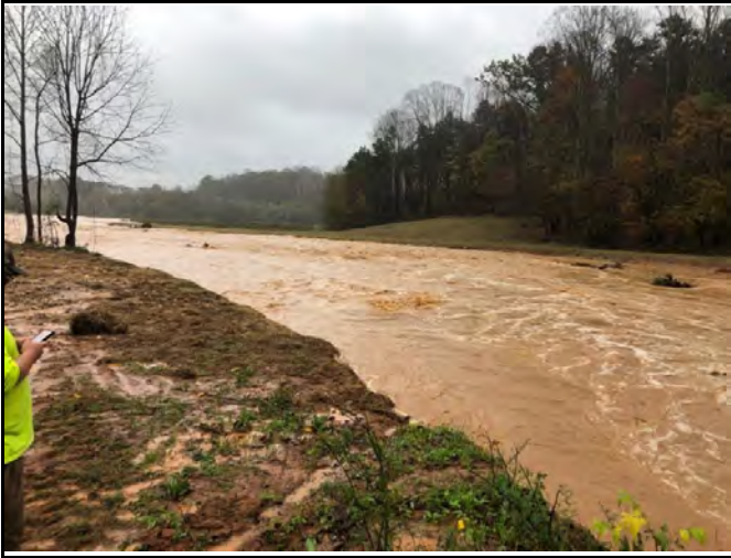
Flooding from Hurricane Zeta remnants on Upper R7 (10/29/20)
