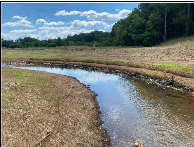
PP-5: Reach 7, downstream, Station 13+75
