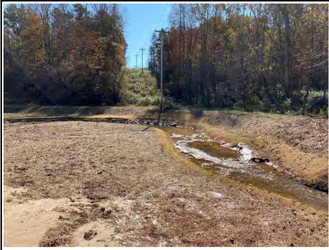
Upper R7 Before Storm (10/14/20)
