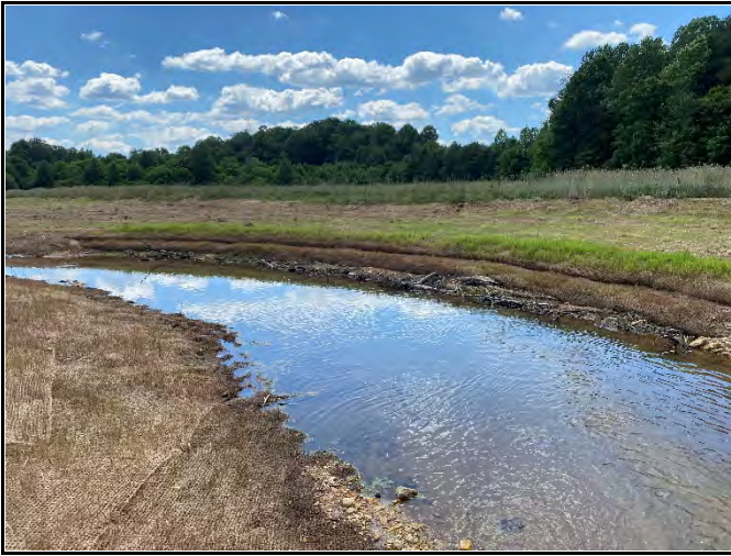
PP-9: Reach 7, downstream, Station 16+00
