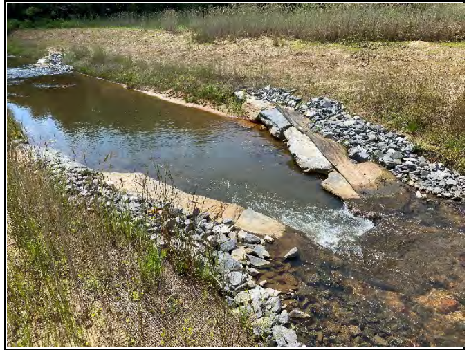
PP-20: Reach 7, downstream, Station 23+25
