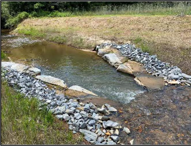
PP-21: Reach 7, downstream, Station 24+00
