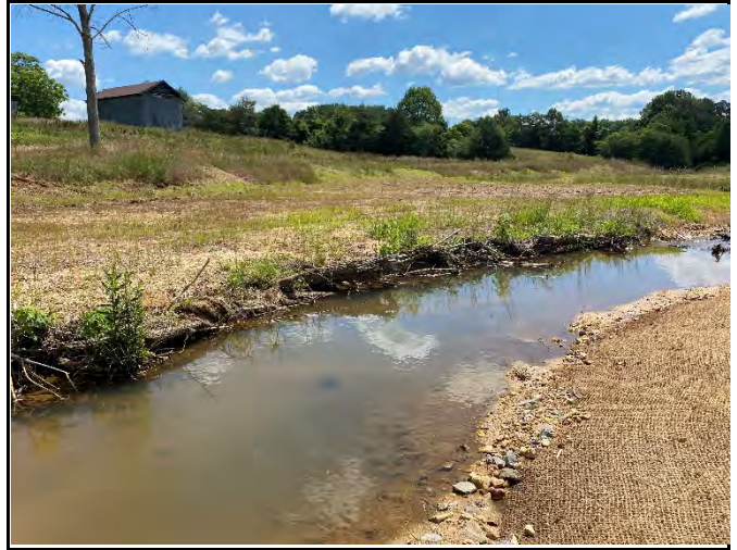
PP-14: Reach 7, downstream, Station 19+25
