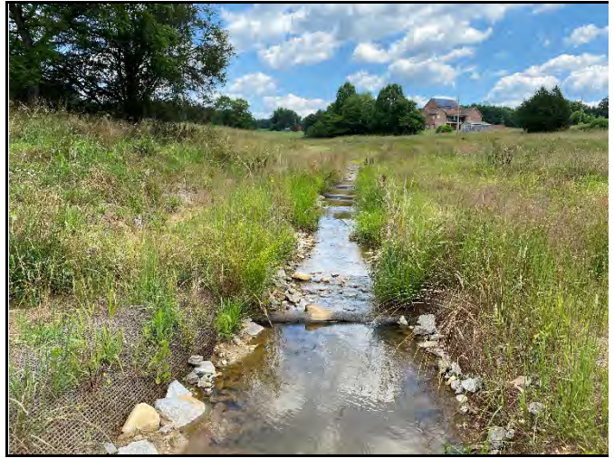
PP-40: Reach UT5, upstream, Station 16+15
