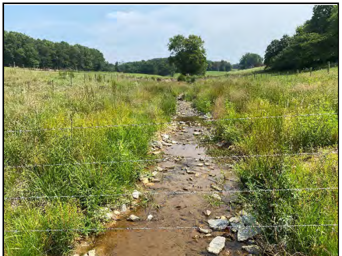
UT5 Rock Ford Crossing after fencing/gates installed, looking upstream with interior wire (7/22/21)
