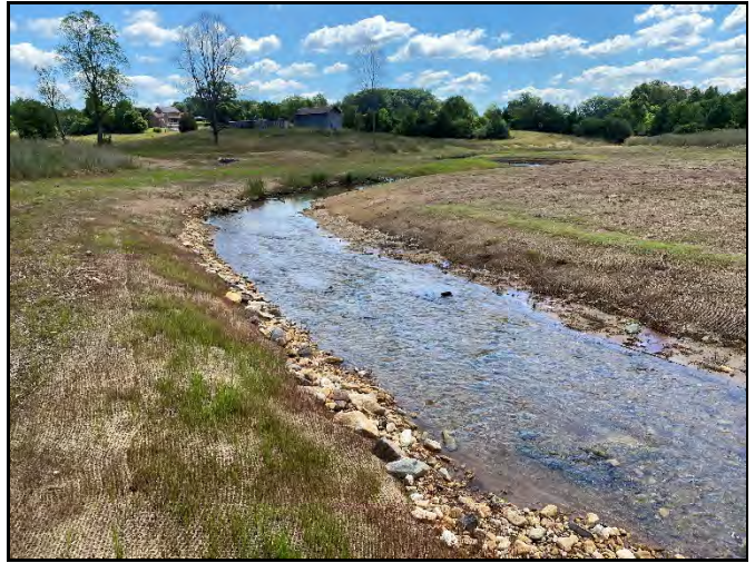
PP-10: Reach 7, downstream, Station 16+50
