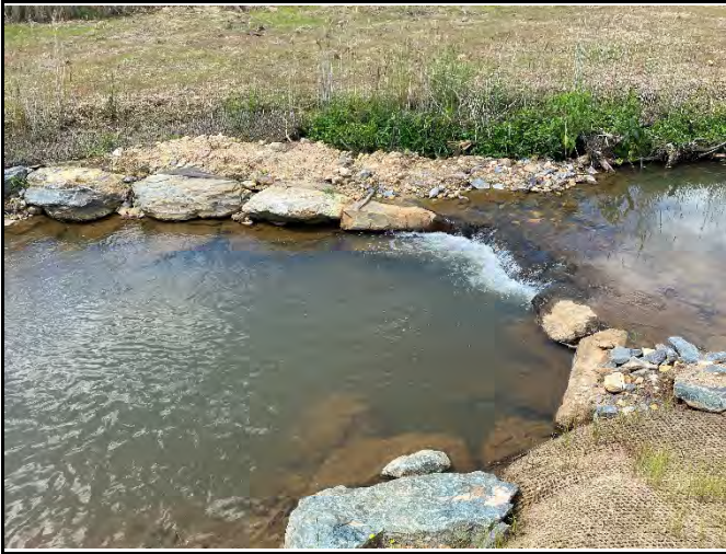
PP-19: Reach 7, upstream, Station 22+75
