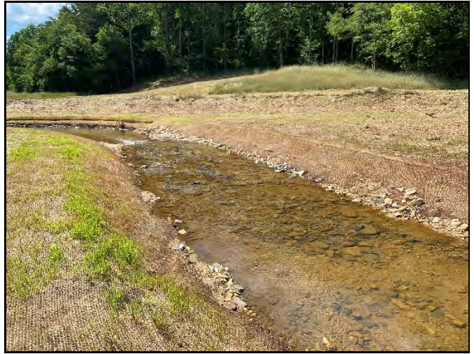
PP-4: Reach 7, downstream, Station 13+25
