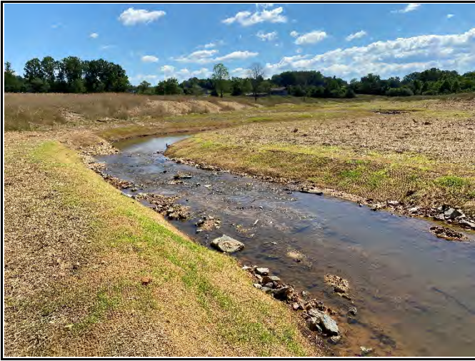
PP-3: Reach 7, downstream, Station 12+00
