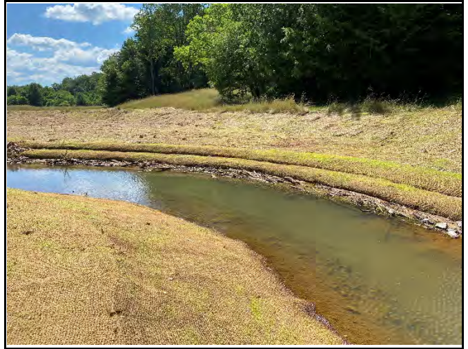
PP-2: Reach 7, downstream, Station 11+00
