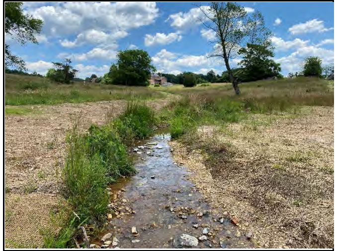
PP-38: Reach UT5, upstream, Station 17+75
