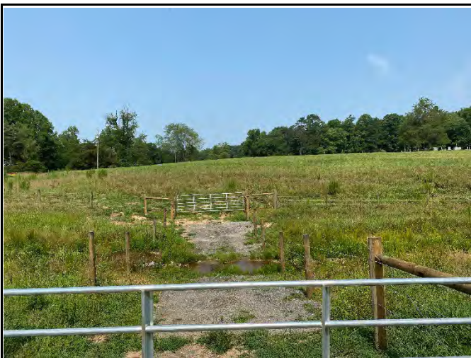
UT5 Rock Ford Crossing after fencing/gates installed (7/22/21)
