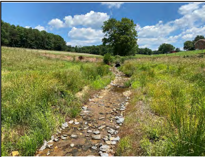
PP-47: Reach UT5, upstream, Station 11+25
