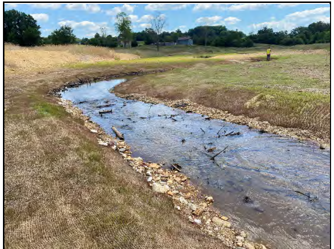
PP-6: Reach 7, downstream, Station 14+25
