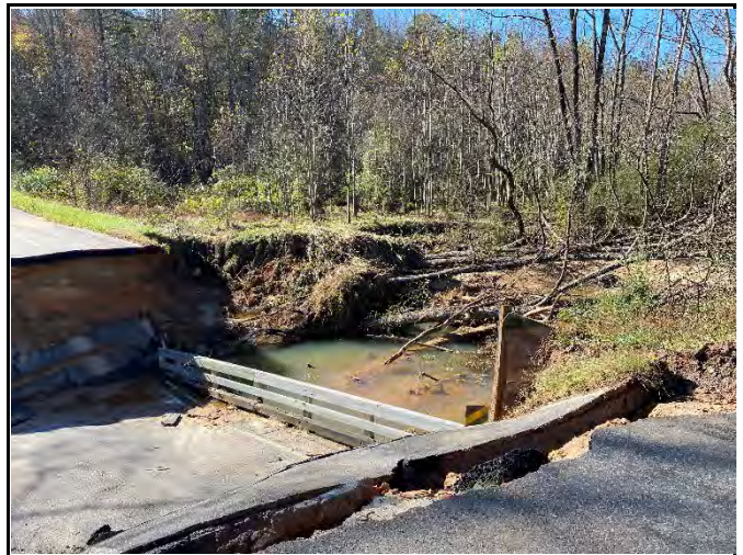
Looking upstream of the bridge (11/4/20)
