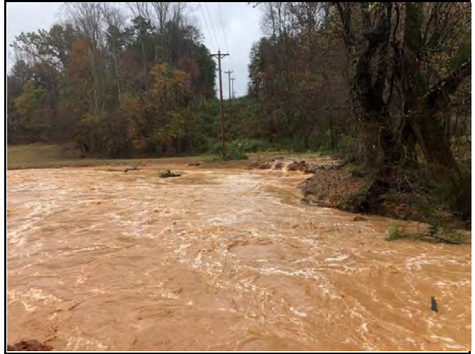
Flooding from Hurricane Zeta remnants on Upper R7 just below bridge (10/29/20)
