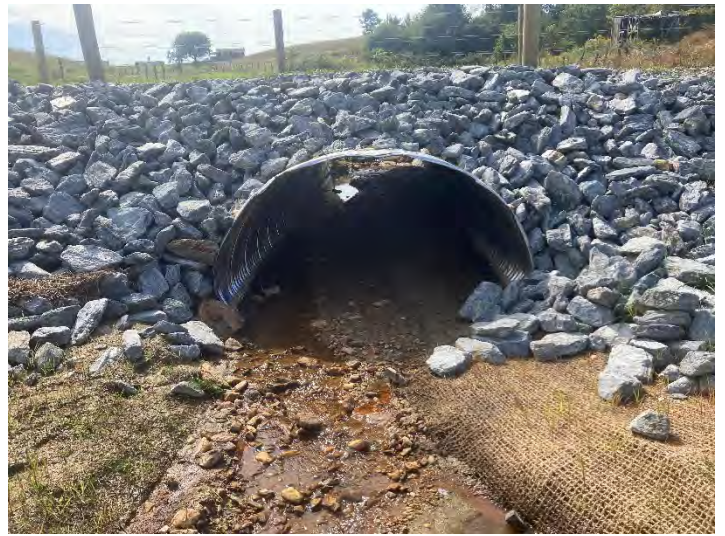
UT to Crab Creek Reach 1 Crossing 1 (103+33) – outlet (9/28/2021)
