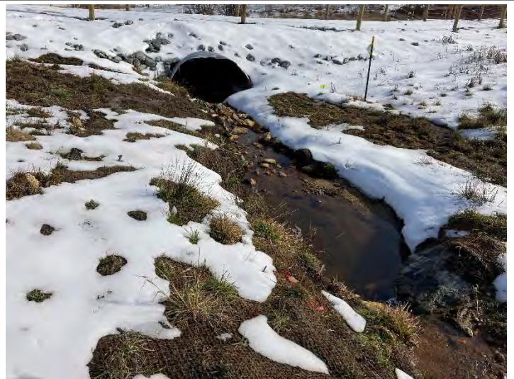
PHOTO POINT 3 UT to CC Reach 1 – downstream (1/25/2022)
