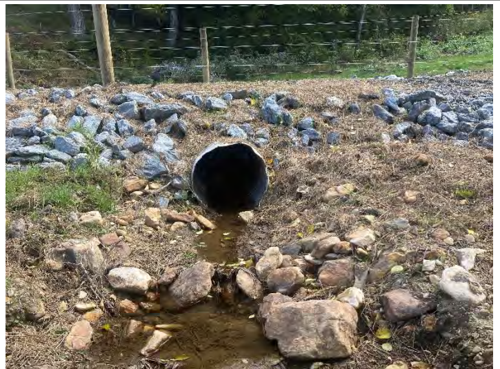
UT6 Crossing (605+71) – outlet (9/28/2021)
