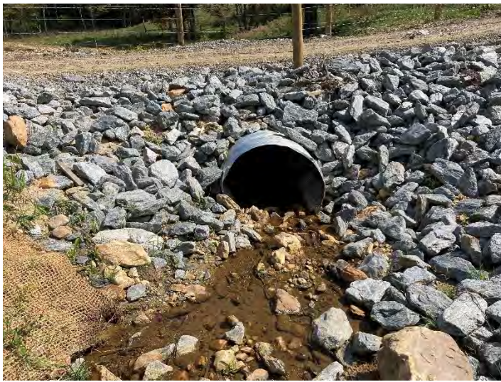
UT4 Reach 2 Crossing (413+54) – inlet (9/29/2021)
