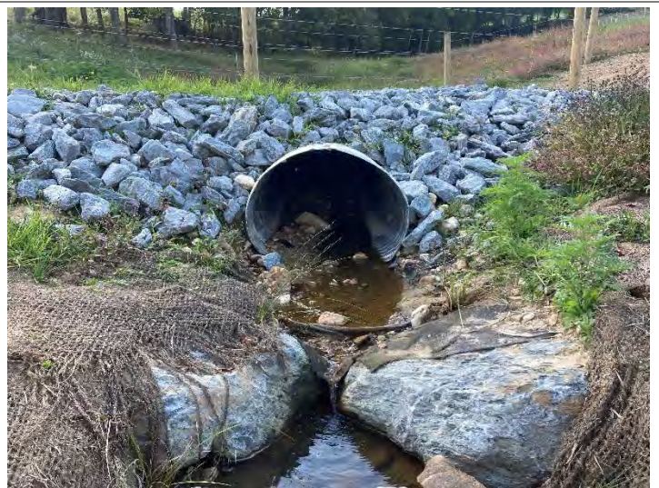
UT1A Reach 1 Crossing (155+17) – outlet (9/28/2021)
