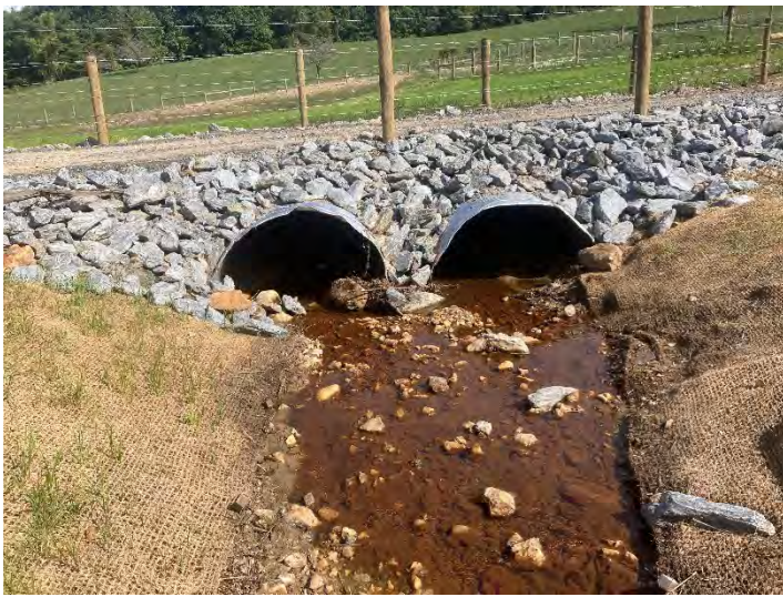
UT to Crab Creek R1 Crossing 2 (114+46) – inlet (9/28/2021)
