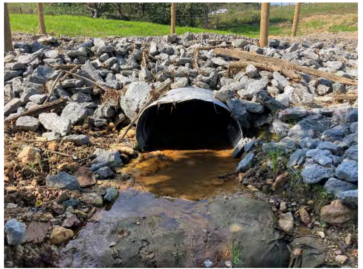
UT4 Reach 2 Crossing (413+96) – outlet (9/29/2021)
