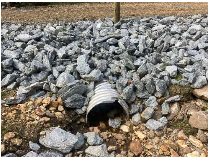
UT6 Crossing (605+26) – inlet (9/28/2021)
