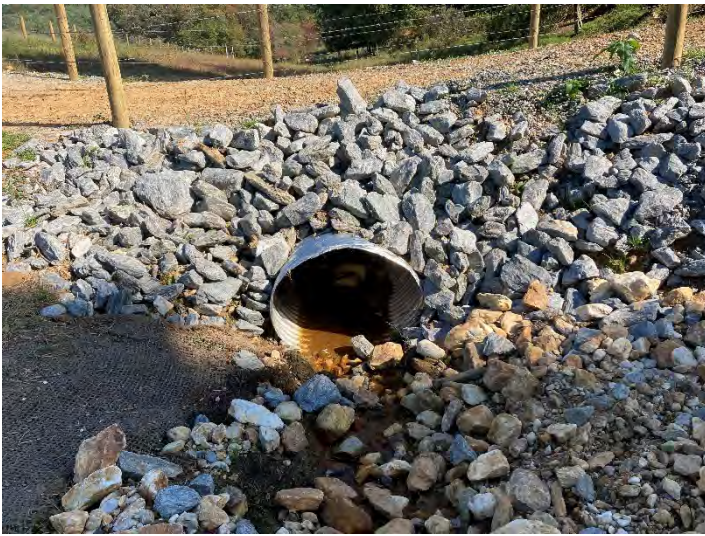
UT4 Reach 1 Crossing (404+33) – inlet (9/29/2021)
