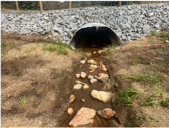
UT to Crab Creek Reach 1 Crossing 1 (102+83) – inlet (9/28/2021)
