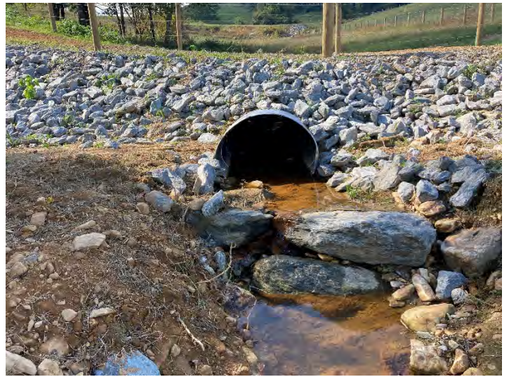
UT4 Reach 1 Crossing (404+74) – outlet (9/29/2021)
