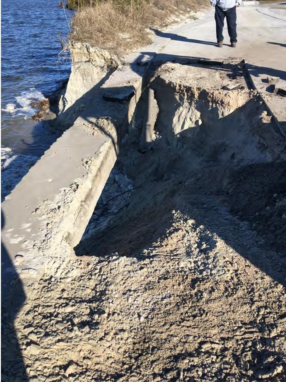
Erosion exacerbated by County improperly capping fire hydrant during removal. January 17, 2020.
