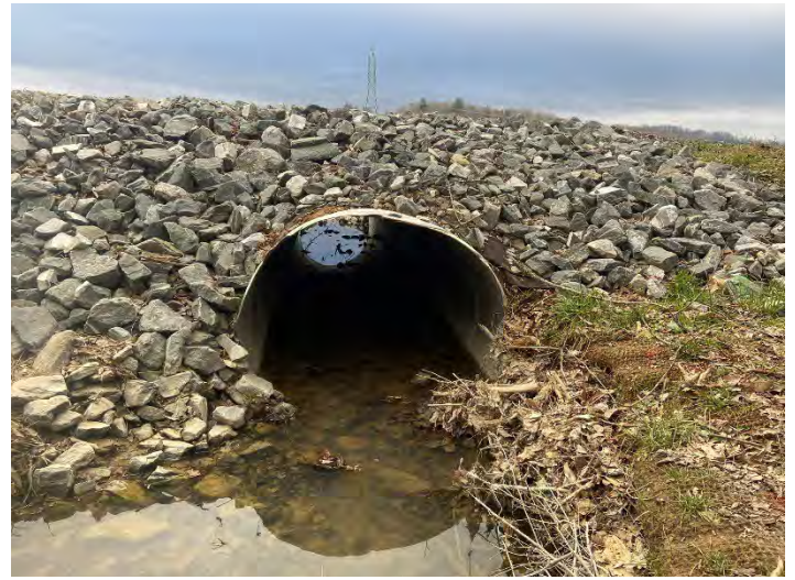
Culvert Crossing – Upper UT1, view downstream (02/16/2022)
