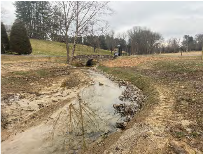
Photo Point 17 – Banner Creek R1, view upstream (02/16/2022)
