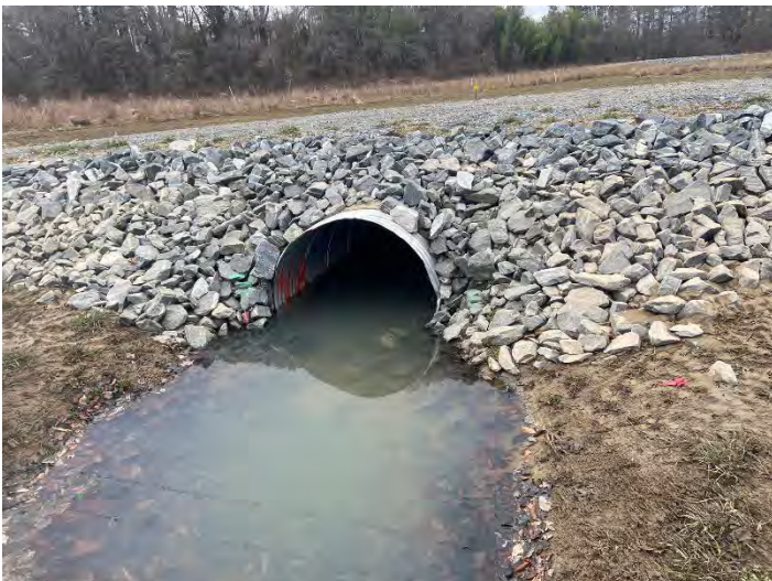
Culvert Crossing – Lower UT1, view upstream (02/16/2022)
