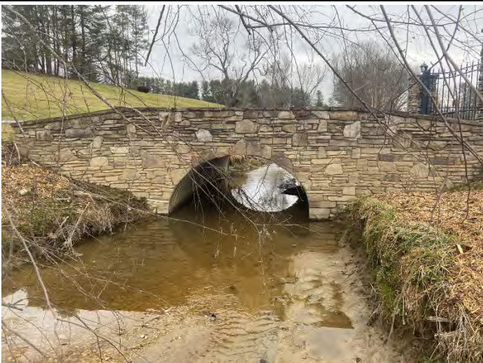
Culvert Crossing – Banner Creek R1, view upstream (02/16/2022)
