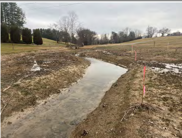
Photo Point 16 – Banner Creek R1, view upstream (02/16/2022)
