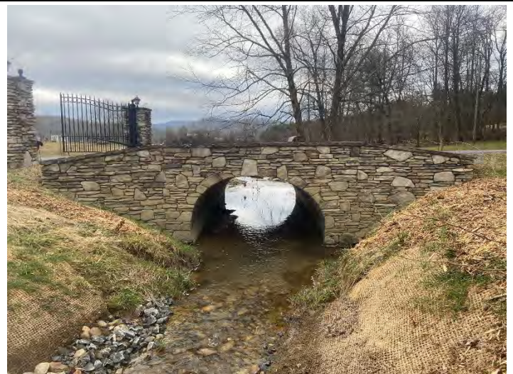
Culvert Crossing – Banner Creek R1, view downstream (02/16/2022)
