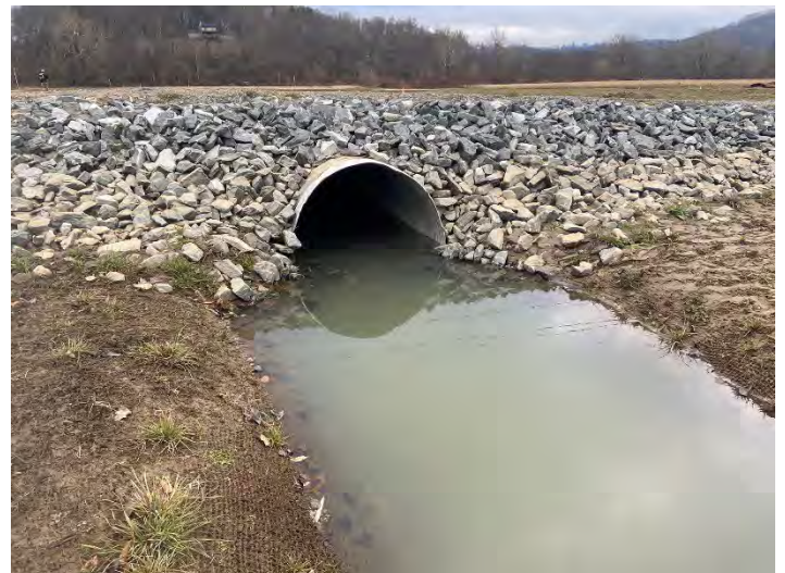
Culvert Crossing – Lower UT1, view downstream (02/16/2022)
