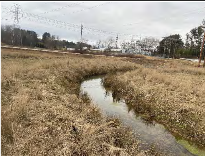
Photo Point 9 – Banner Creek R3, view upstream (02/16/2022)
