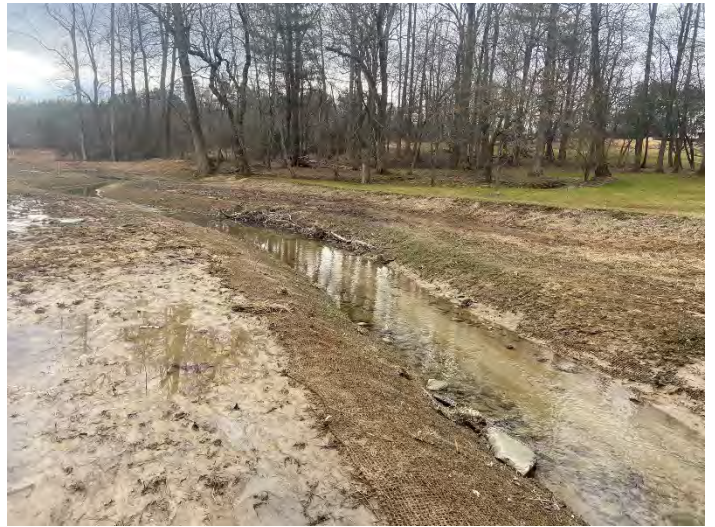
Photo Point 17 – Banner Creek R1, view downstream (02/16/2022)
