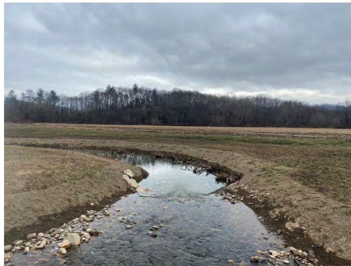
Photo Point 7 – Banner Creek R4a, view downstream (02/16/2022)
