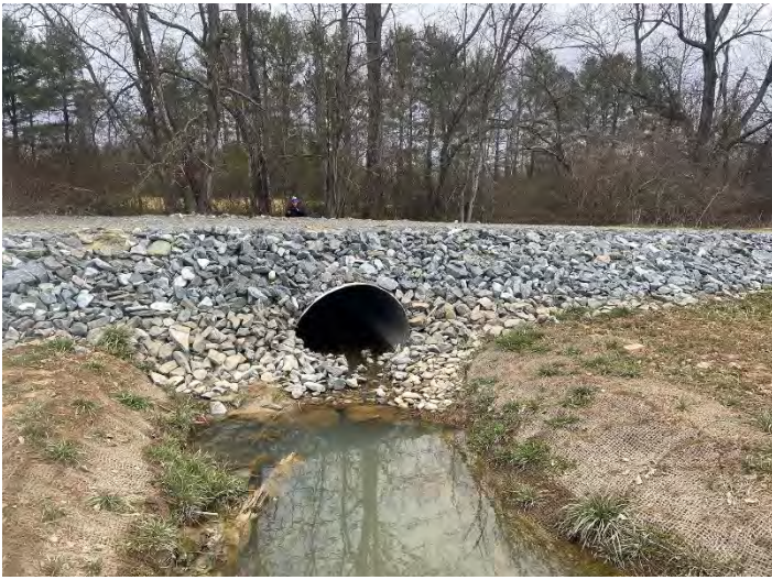
Culvert Crossing – Upper UT1, view upstream (02/16/2022)
