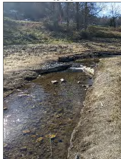
PP-30: R2, Upstream, Station 16+50
