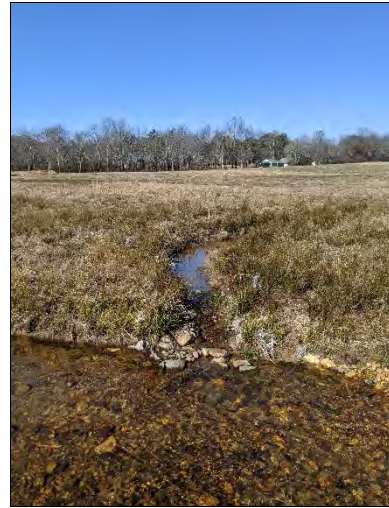
PP-43: R1, Swale on Left Floodplain, Station 17+00
