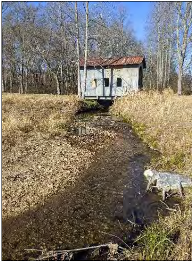
PP-1: R1 Upstream, Station 10+75- Begin R1
