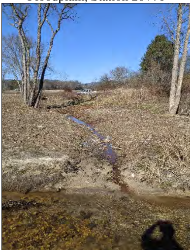
PP-46: R1, Overflow Channel on Left Floodplain, Station 26+75
