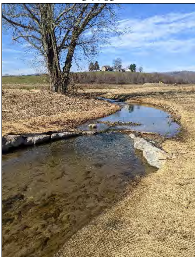
PP-23: R1, Upstream, Station 37+00 – End R1
