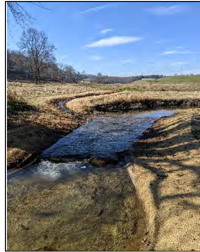
PP-22: R1, Upstream, Station 36+75
