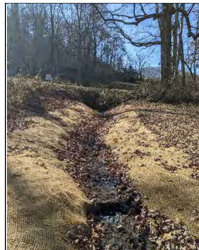
PP-24: UT1, Upstream, Station 10+60
