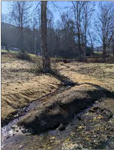
PP-25: UT1, Upstream, Station 11+85- Confluence with R2
