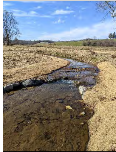
PP-38: R2, Upstream, Station 24+60
