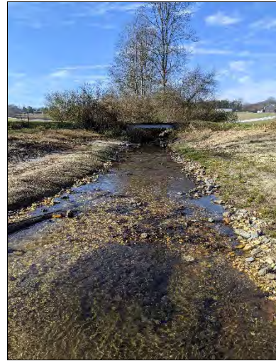
PP-26: R2, Upstream, Station 10+50- Begin R2
