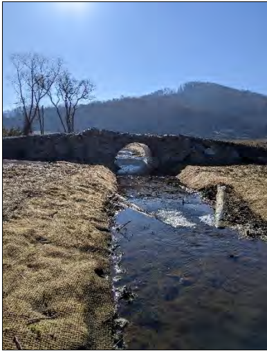
PP-13: R1, Downstream, Station 24+25- Culvert
