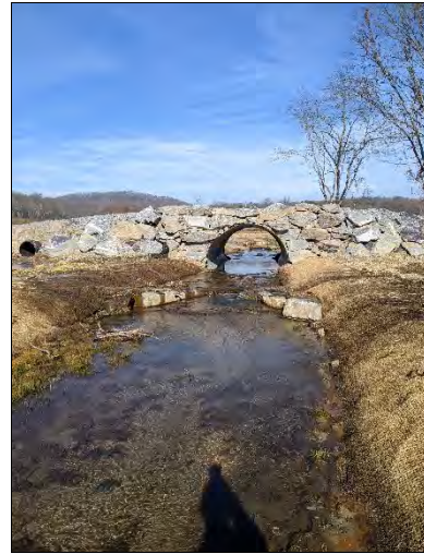
PP-14: R1, Upstream, Station 25+60- Culvert
