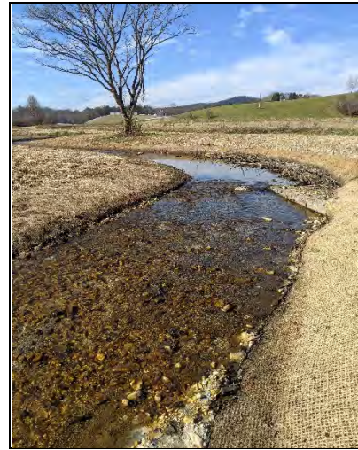
PP-34: R2, Upstream at Station 20+80
