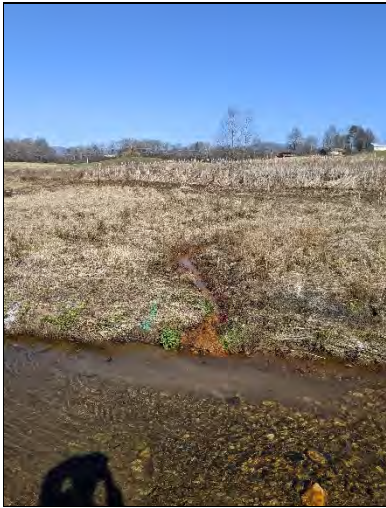
PP-44: R1, Swale on Left Floodplain, Station 20+70
