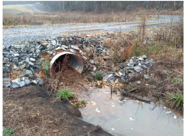
PHOTO POINT 4 - Carpenter Bottom R1 - downstream (2/3/2022)
