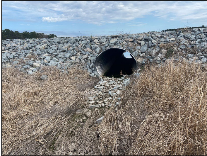
Culvert at the top of KJ1-C (3/8/2022)
