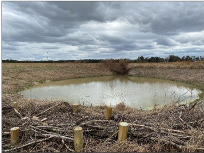
ESP & Treatment Pool (3/16/2022)
