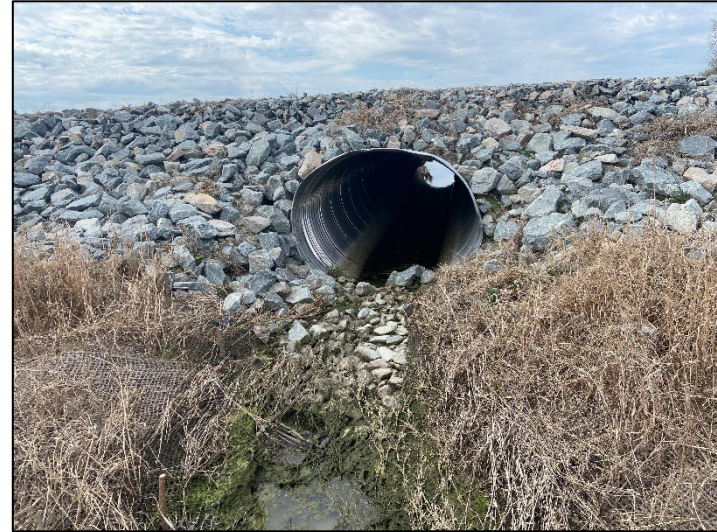
Culvert at the bottom of KJ1-B (3/8/2022)
