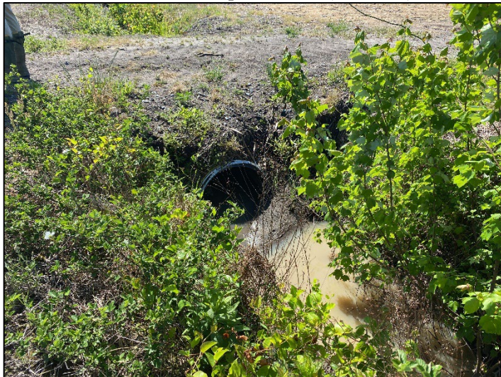
Culvert at edge of Wetland (4/28/2022)
