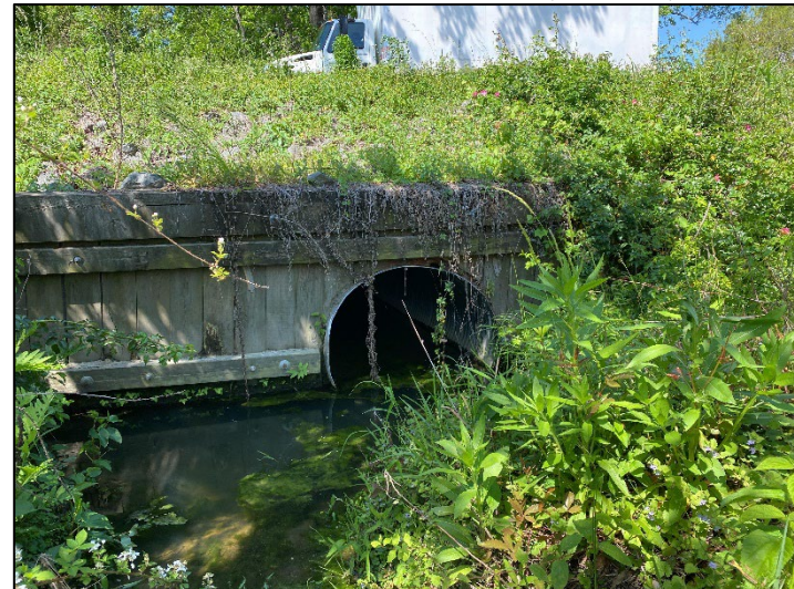
Culvert at Kinston Highway (4/28/2022)
