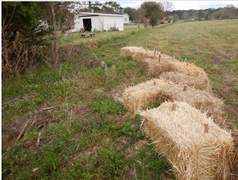
Erosion Control and Reduction Via Live Stakes and Sheet Flow Diversion (4/5/2022)
