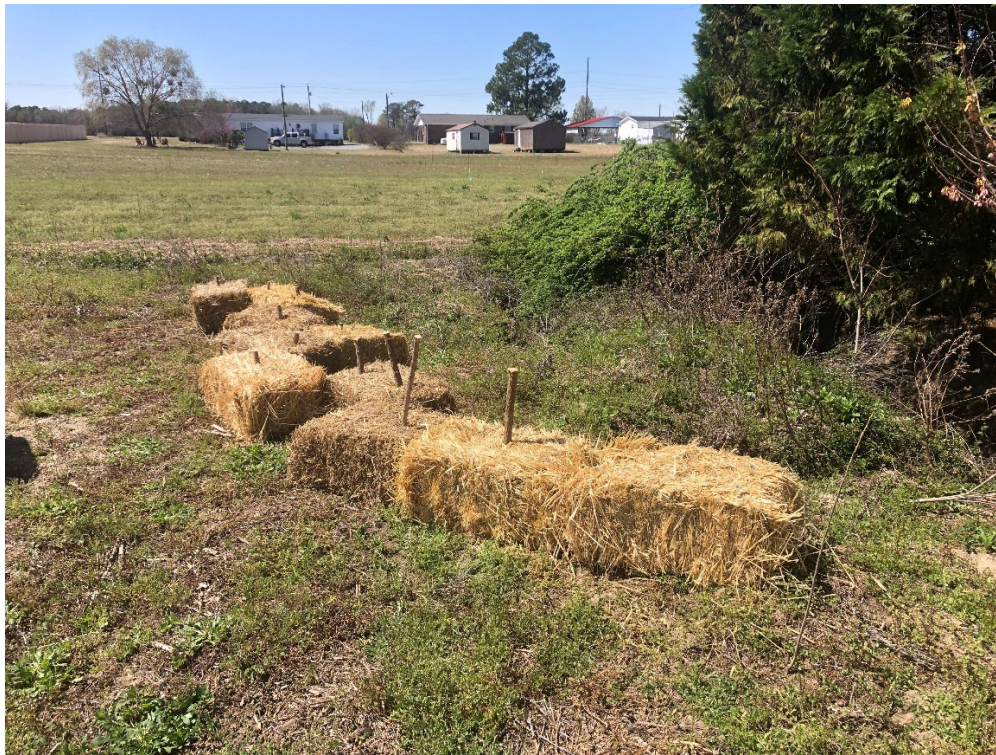
Erosion Control and Reduction Via Live Stakes and Sheet Flow Diversion (3/29/2022)
