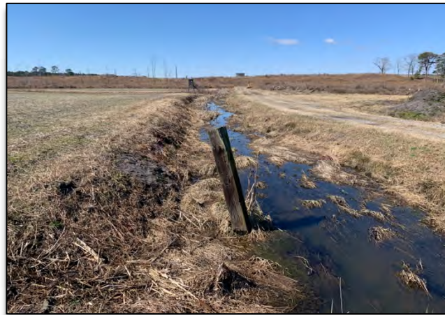
West view of Main West-East Ditch.
