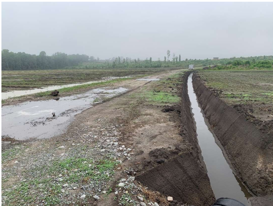
Constructed Drainage Ditch North of the Site (view west) – taken 5/25/2022
