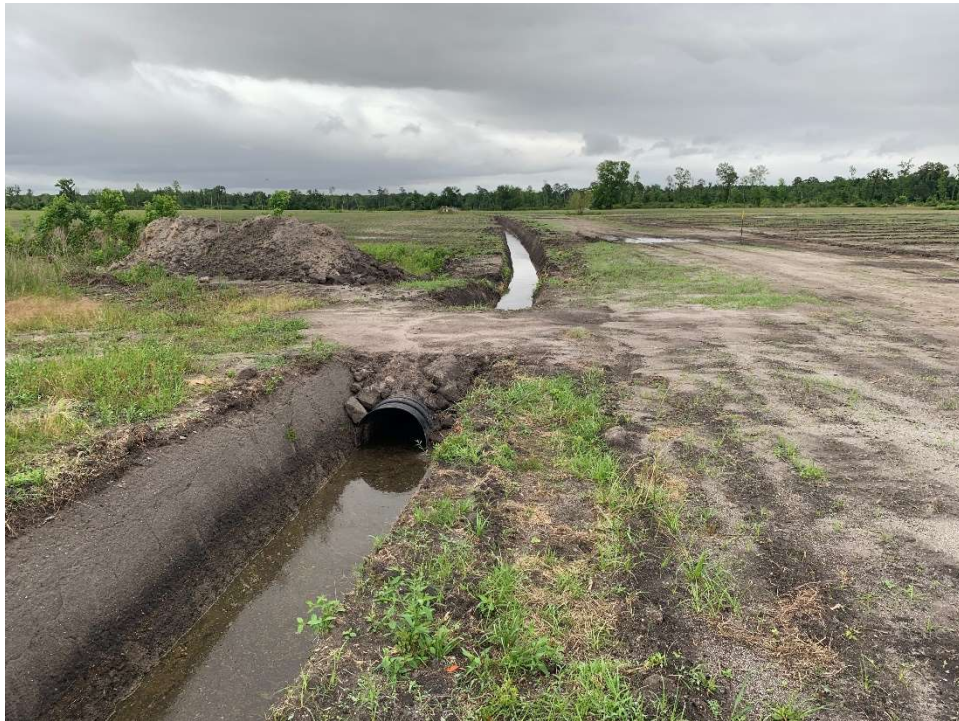
Constructed Drainage Ditch North of the Site (view east) – taken 5/25/2022
