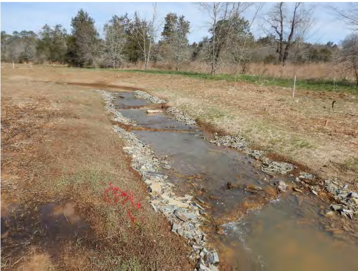
PHOTO POINT 5 UT1 R1 – upstream (03/13/2022)
