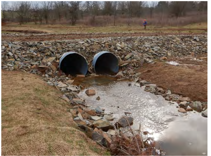
UT1B - Looking Downstream (02/08/2022)
