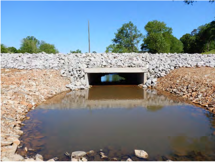
UT1 R2 - Looking Upstream (05/09/2022)
