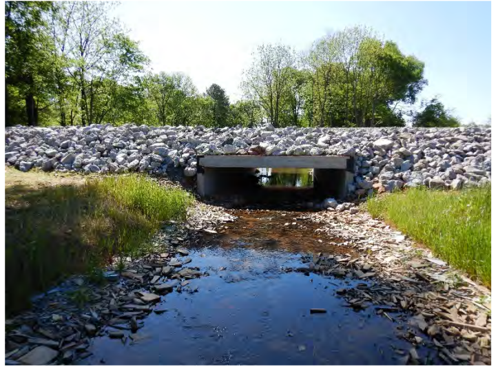
UT1 R2 - Looking Downstream (05/09/2022)
