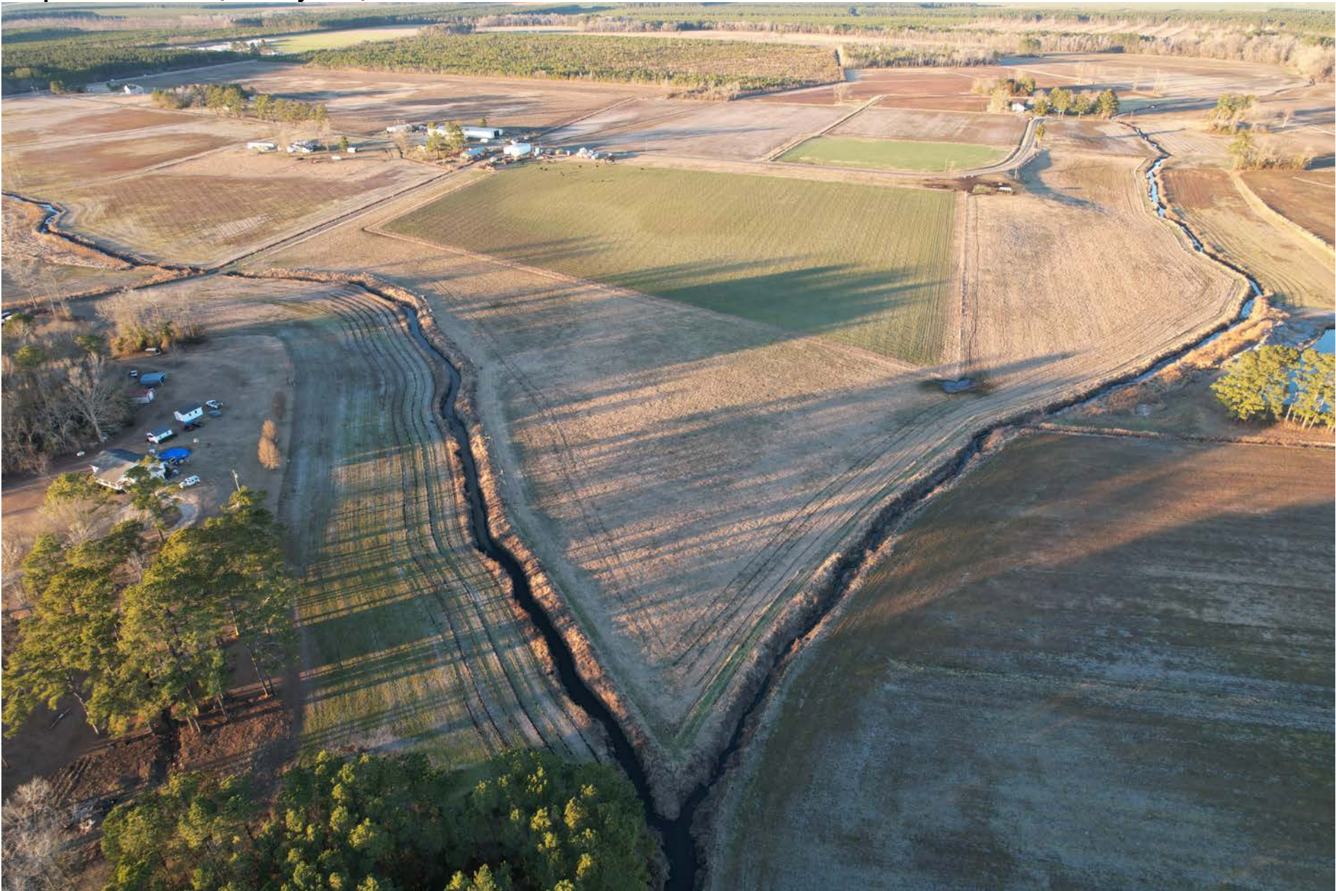
Site post construction (February 2022)
