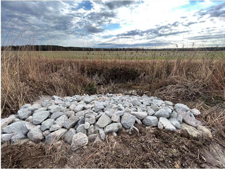
Ditch Plug at Southeastern Site Boundary (Ditch A) – view east
