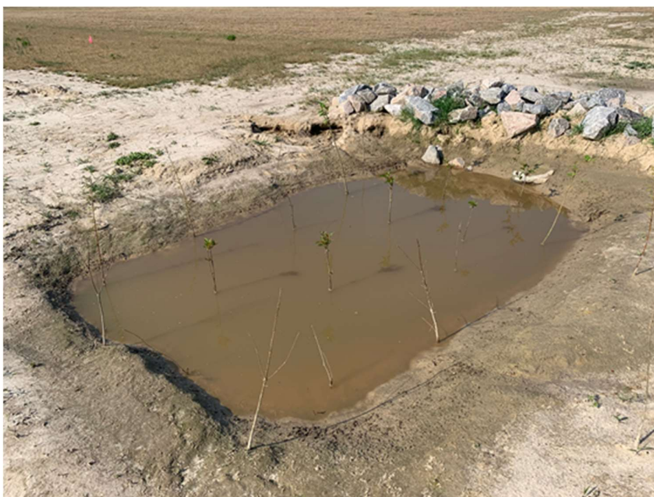
Southernmost Ditch Plug with Sediment Forebay on Western Site Boundary – view southwest
