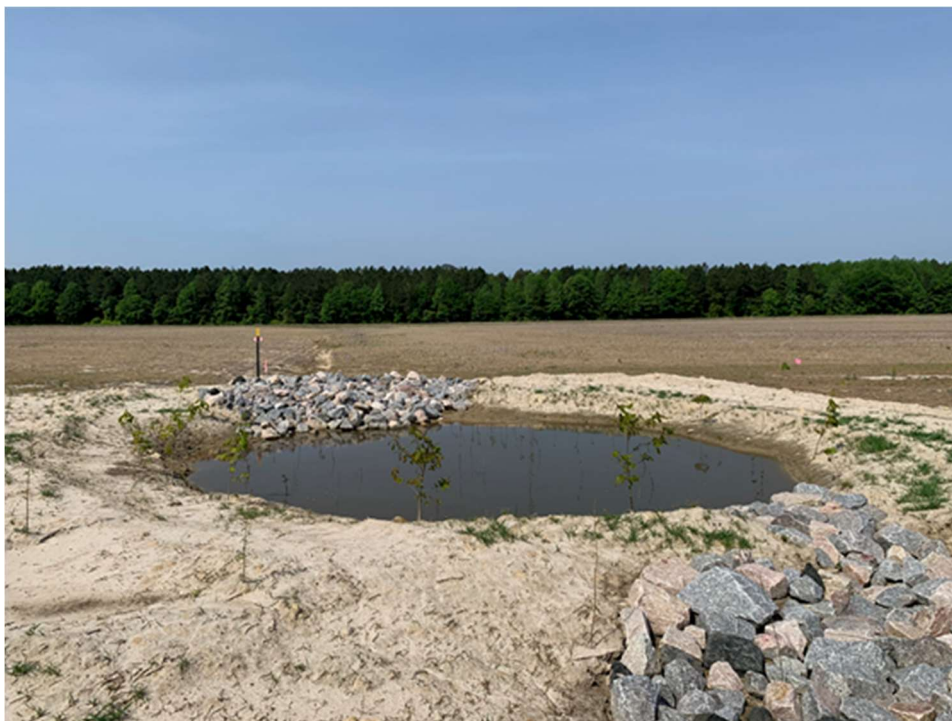
Northernmost Ditch Plug with Sediment Forebay on Western Site Boundary – view west
