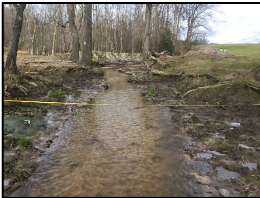
Looking upstream along reach DE4-B, DS of the culvert crossing
