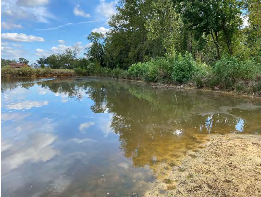
Photo 1: Upstream face of the dam taken from western shore, looking east.
