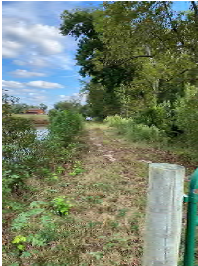
Photo 2: Upstream face with defined tire tracks along dam crest, looking east.
