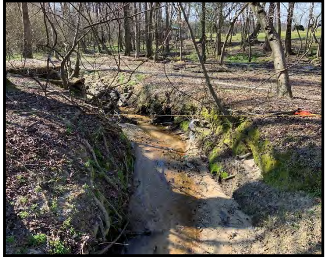
Brad's Branch below Darden Road
