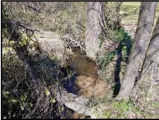
Looking upstream along reach DE4-B, US of the culvert crossing
