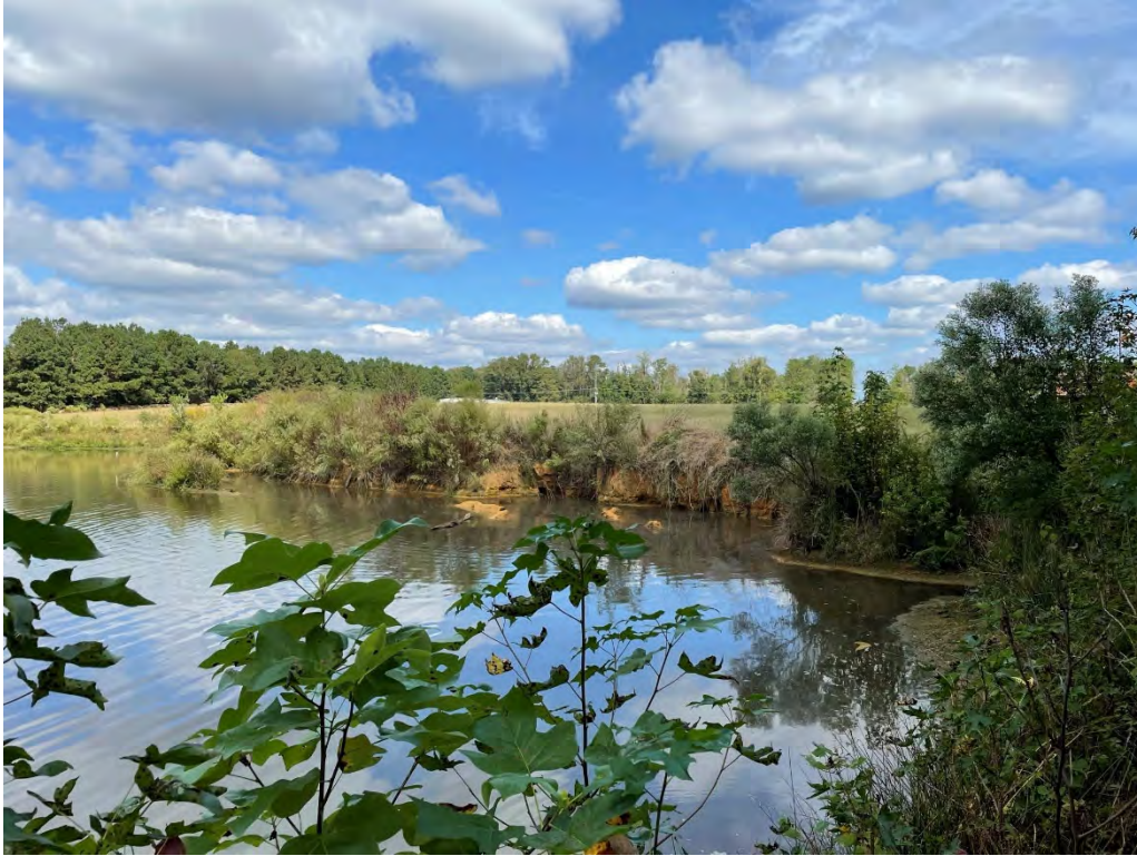
Photo 3: Vertical bank sloughing in vicinity of outfall pipe (hidden at right), looking northeast.
