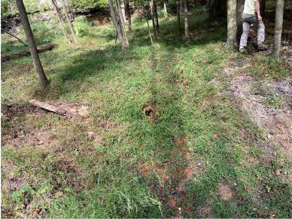
Photo 13: Shallow channel about 75-100 feet from downstream toe of dam.
