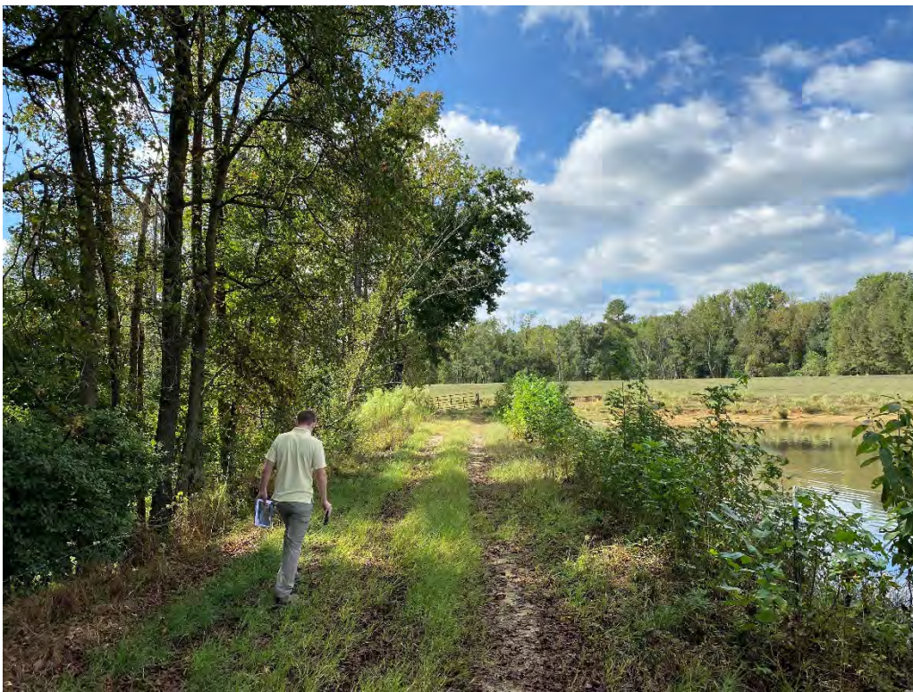
Photo 4: Dam crest looking west.
