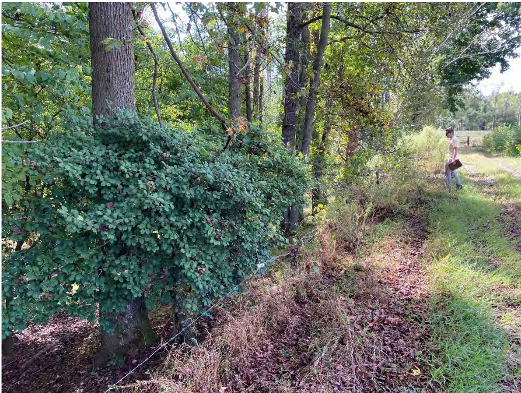
Photo 6: Downstream face heavily vegetated by trees, looking west.
