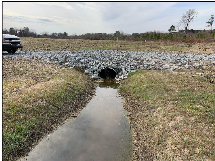
Culvert at JH1-B Crossing (Entrance) (3/7/2022)
