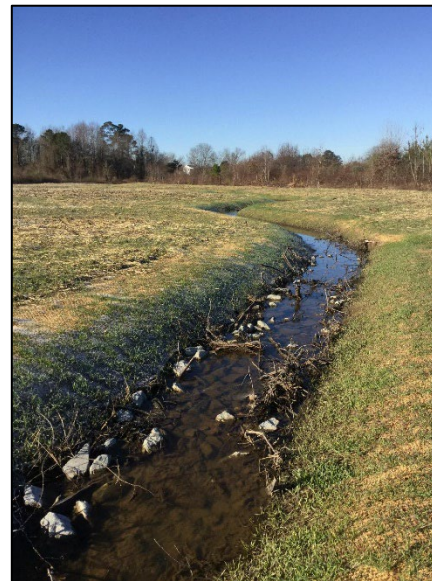
Wood/rock riffle – JH1-B (3/15/2022)
