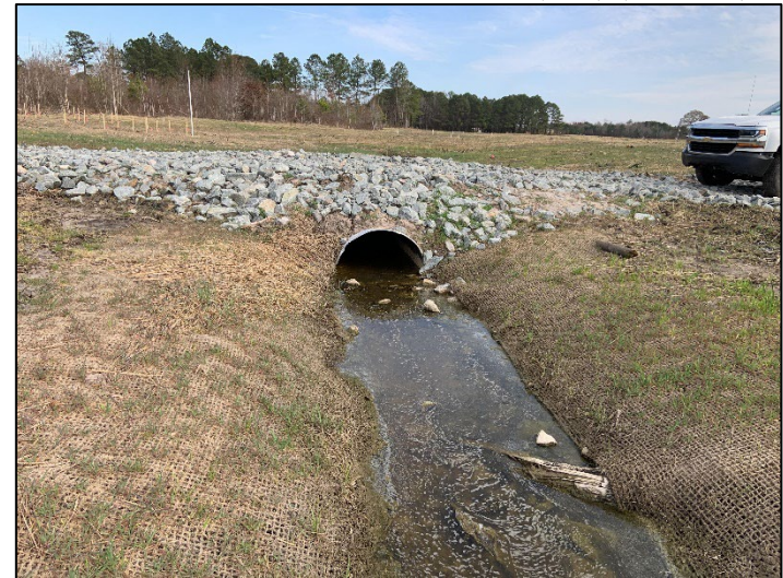
Culvert at JH1-B Crossing (Exit) (3/7/2022)
