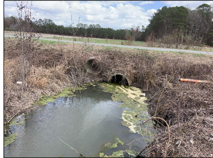
DOT Culvert at Yelverton Grove Rd. (Exit) (3/7/2022)
