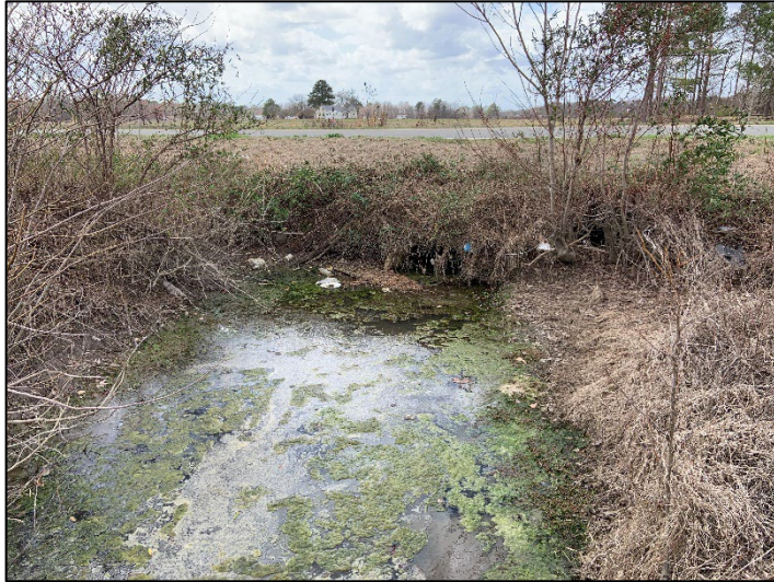
DOT Culvert at Yelverton Grove Rd. (Entrance) (3/7/2022)
