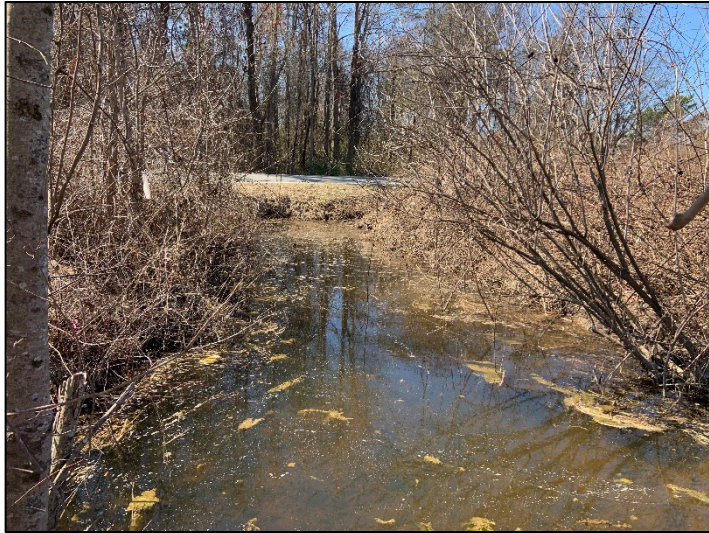
DOT Culvert at Brogden Rd. (Entrance) (3/7/2022)
