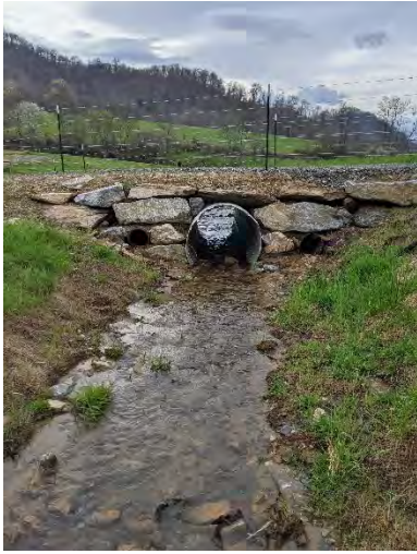
PP-43: UT3, Station 22+15. Facing Downstream.
