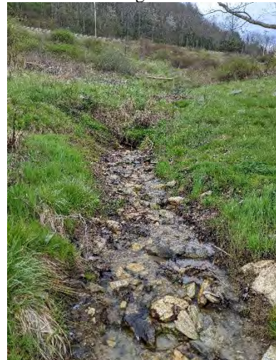
PP-30: UT3, Station 10+00. Facing Upstream.
