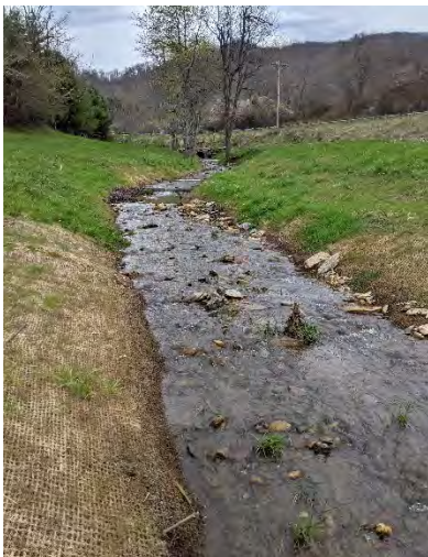
PP-51: UT1, Reach 4, Station 33+10. Facing Upstream.
