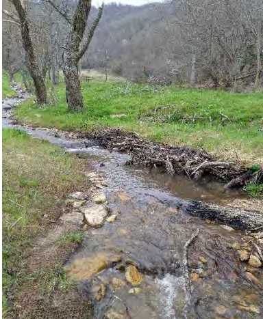
PP-13: UT1, Reach 3, Station 18+90. Facing Upstream.
