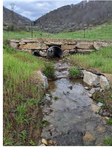
PP-44: UT3, Station 23+15 Facing Upstream.
