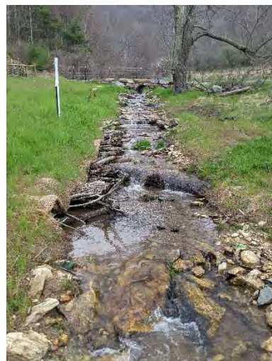
PP-7: UT1, Reach 2, Station 14+60. Facing Upstream.
