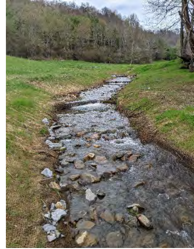
PP-56: UT1, Reach 4, Station 37+00. Facing Upstream.
