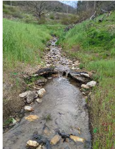
PP-32: UT3, Station 11+75. Facing Upstream.
