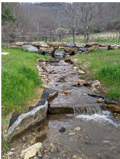
PP-6: UT1, Reach 2, Station 13+25. Facing Upstream.
