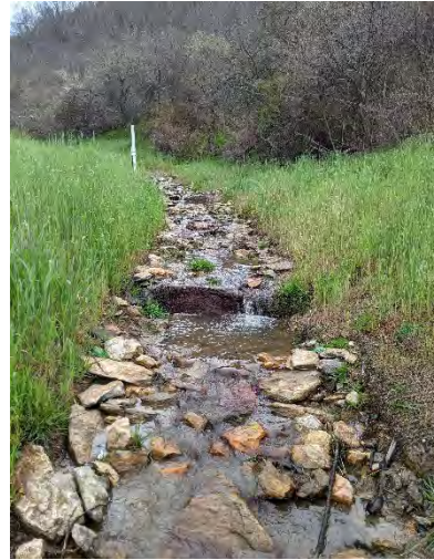
PP-34: UT3, Station 14+15. Facing Upstream.
