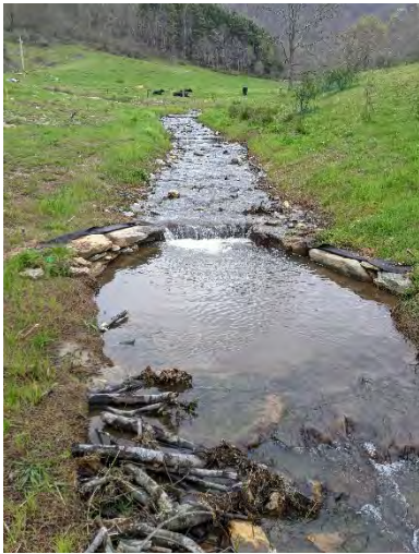
PP-21: UT1, Reach 4, Station 23+90. Facing Upstream.
