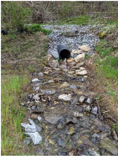
PP-15: UT2, Station 10+15. Facing Upstream.
