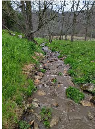
PP-8: UT1, Reach 2, Station 15+50. Facing Upstream.
