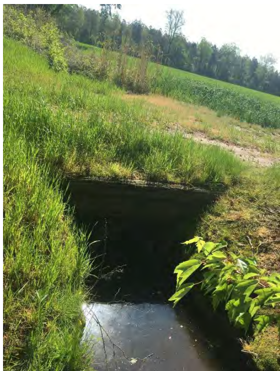
6. Ditch 1, looking upstream (east) from stream dam
