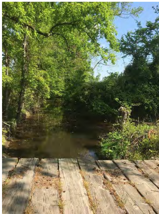
8. Crossing above site, showing inundation from beaver dam.
