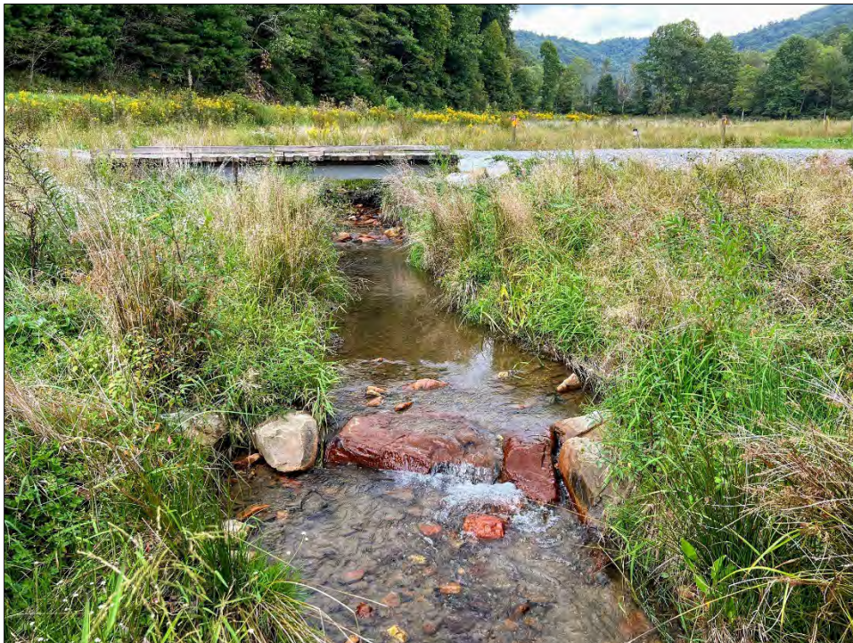
Fork Creek – Rock sill, typical – August 25, 2022
