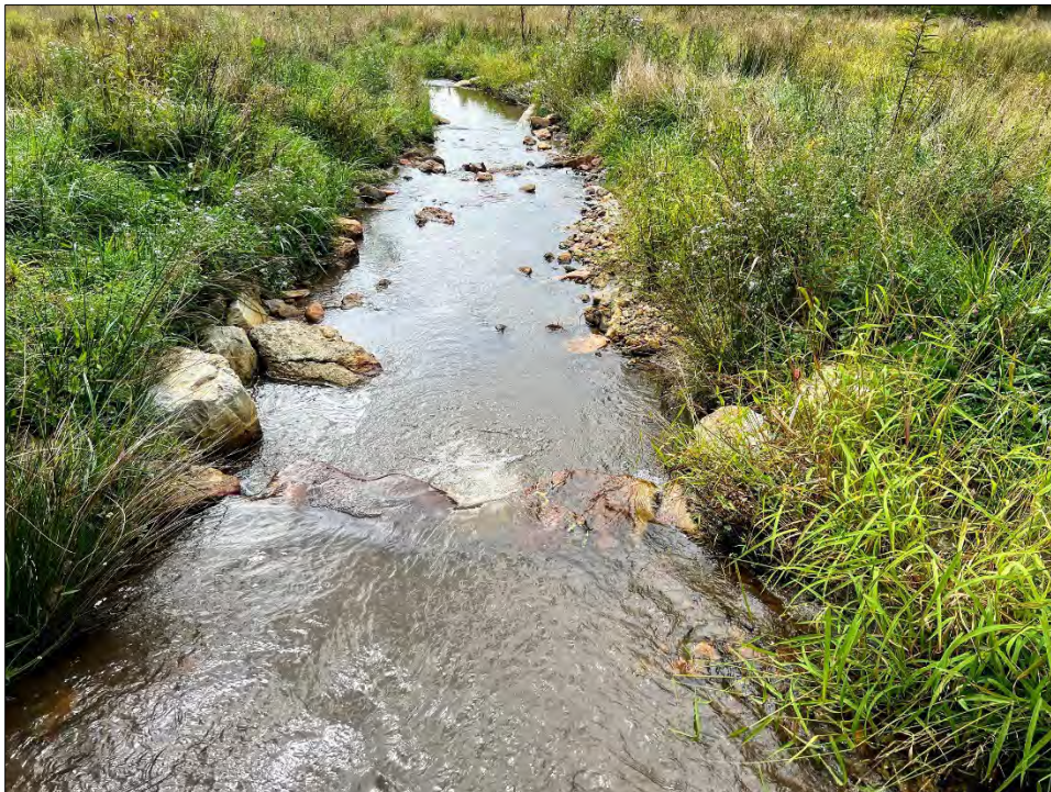
Fork Creek – Rock sill, typical – August 25, 2022
