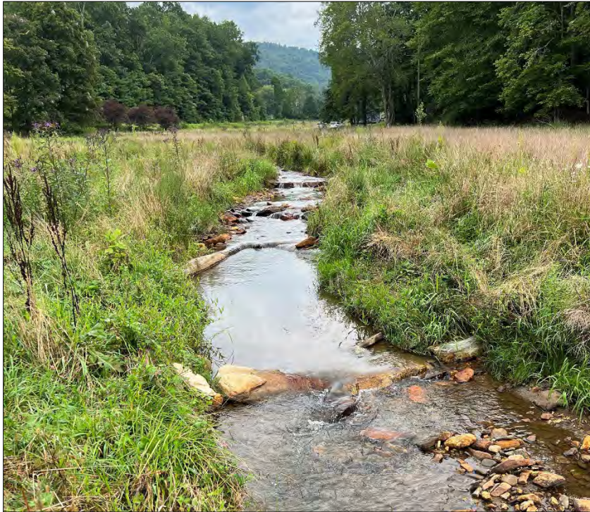
Fork Creek – Rock sill, typical – August 25, 2022
