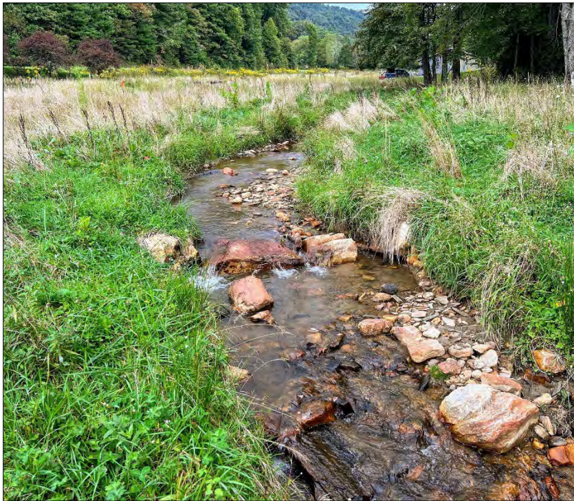
Fork Creek – Rock sill, typical – August 25, 2022
