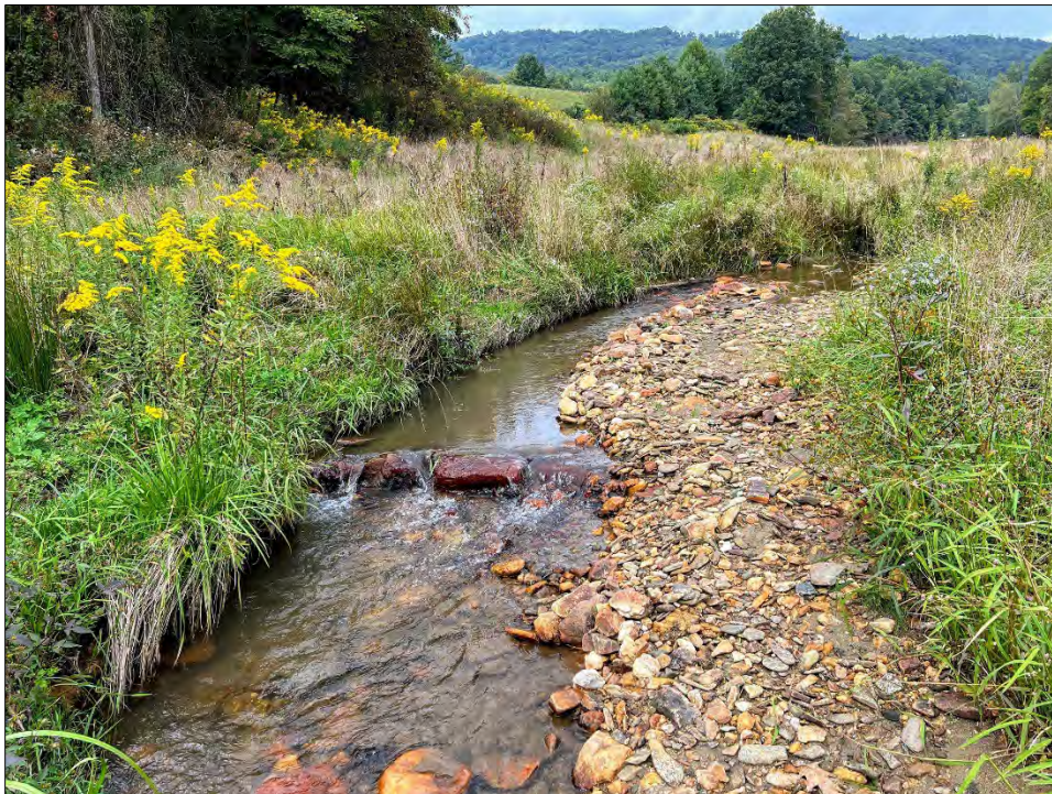
Fork Creek – Rock sill, typical – August 25, 2022
