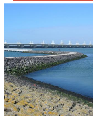
Oosterscheldekering sea wall, the Netherlands
