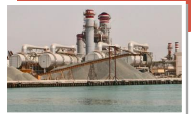
Desalination Plant, United Arab Emirates © Ryan Lackey / Flickr
