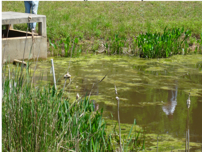
Figure 9-11 Outlet Structure Near Wetland Edge, Orifice Easily Accessible for Maintenance
