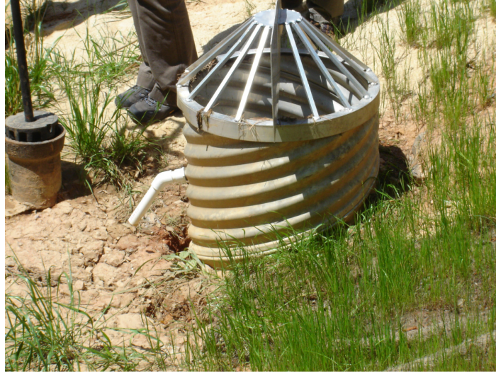
Figure 9-10 Outlet Structure With Down-Turned Drawdown Orifice
