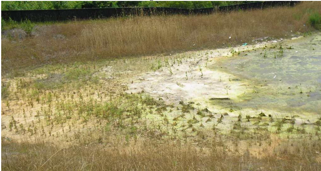
Figure 9-5 Failure to Maintain PPE at Design Elevation in Wetland (Garner, NC)
