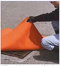
When vehicle washing is performed in the vicinity of a storm drainage collection system, cover the storm drain with a portable drain cover to prevent illegal discharges.
