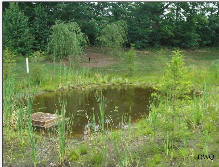
Constructed wetlands are designed similarly to wet ponds but include shallow water, inundation zones, and deep pools. Grading the wetland in zones promotes the growth of wetland vegetation which enhances this BMP's effectiveness. Site areas that are frequently wet or contain pooled water after storm events are usually suitable for a constructed wetland as long as jurisdictional wetlands do not already exist.
