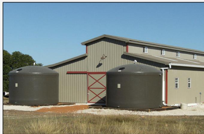
Rainwater is usually drained from a roof to a cistern. Other methods of harvesting rainwater include diverting runoff to a pond where it can be stored and used as needed. This may be more appropriate where larger volumes of water are required only occasionally. Stormwater reuse has additional benefits in that it results in no discharge to receiving waters.
