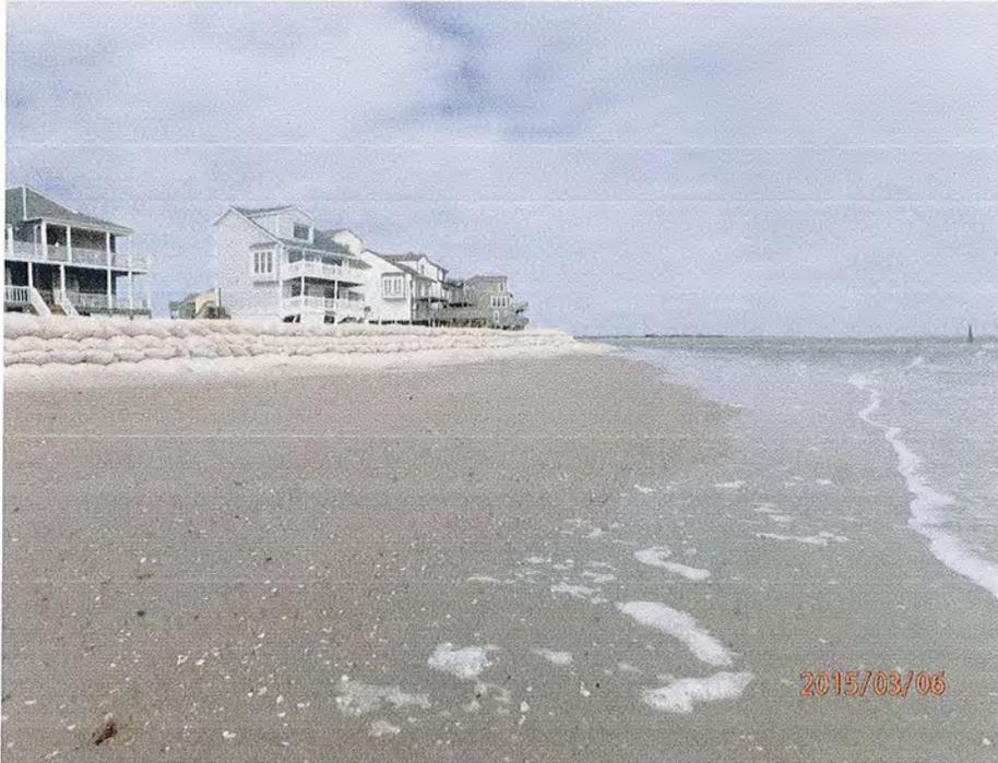
Figure 4. March 6, 2015 photo of sandbag revetment and partially buried sand tube.
