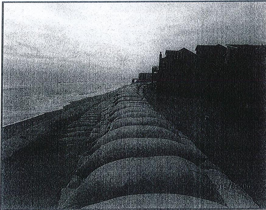
Figure 6. March 6, 2015 photo of sandbag revetment and partially buried sand tube near middle of sandbag revetment.
