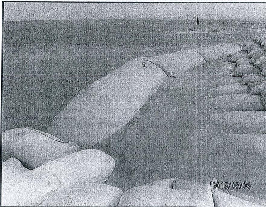
Figure 4. March 6, 2015 photo of sandbag revetment and sand tube at north end of revetment.
