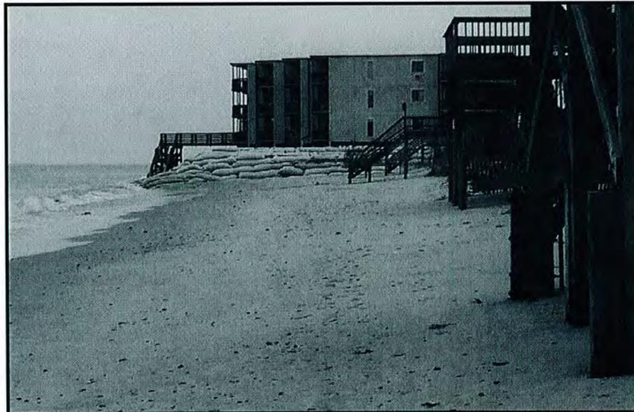
**Photo 8. Sandbags revetment at Topsail Reefs Building 1 (Sep 2014).**
