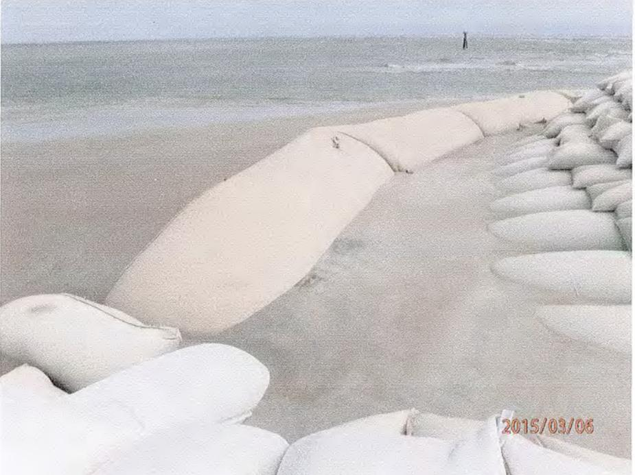
Figure 3. March 6, 2015 photo of sandbag revetment and sand tube at north end of revetment.
