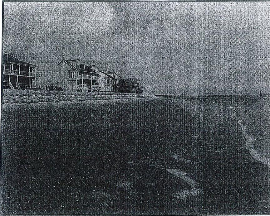
Figure 5. March 6, 2015 photo of sandbag revetment and partially buried sand tube.
