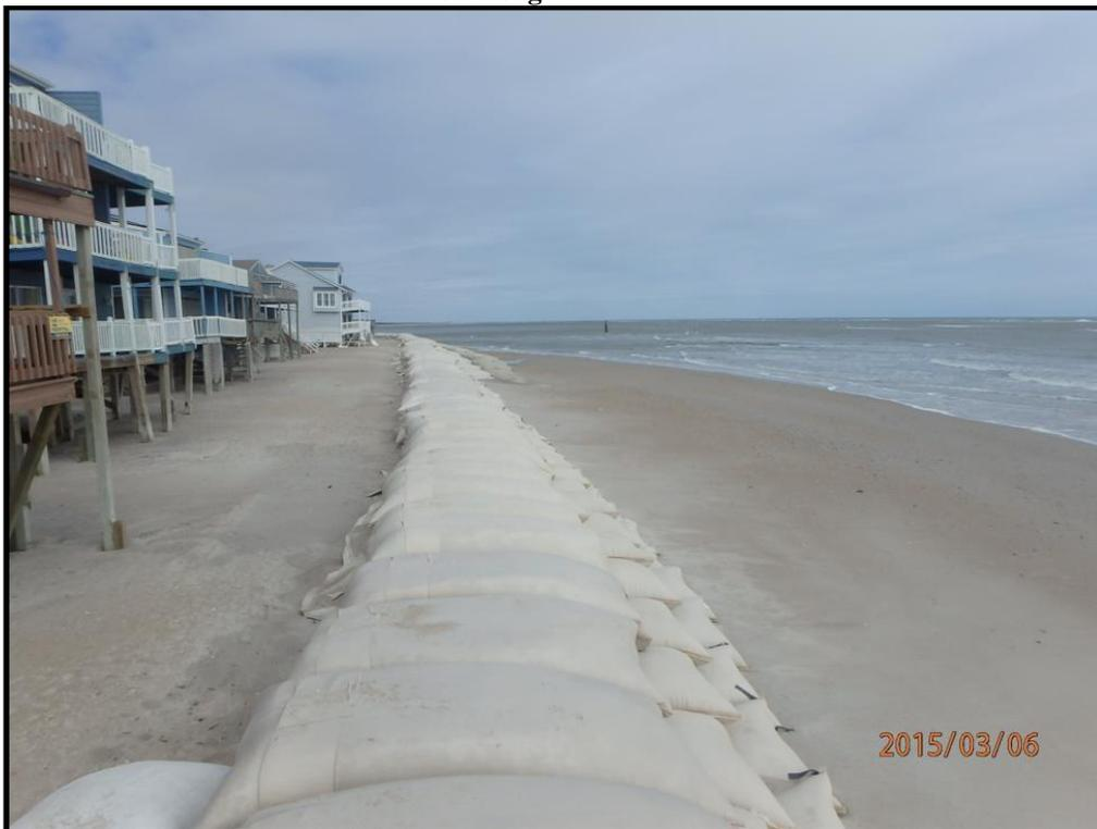
**Figure 7 – March 6, 2015 photo showing buried sand tube along south end of sandbag revetment.**
