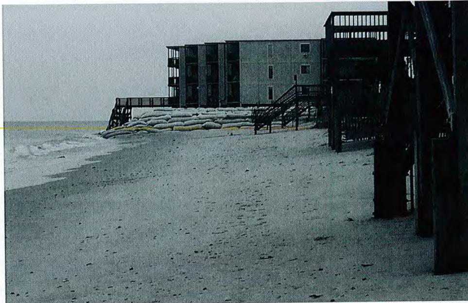
Figure 2. Sandbags revetment at Topsail Reefs Building 1 (Sep 2014).
