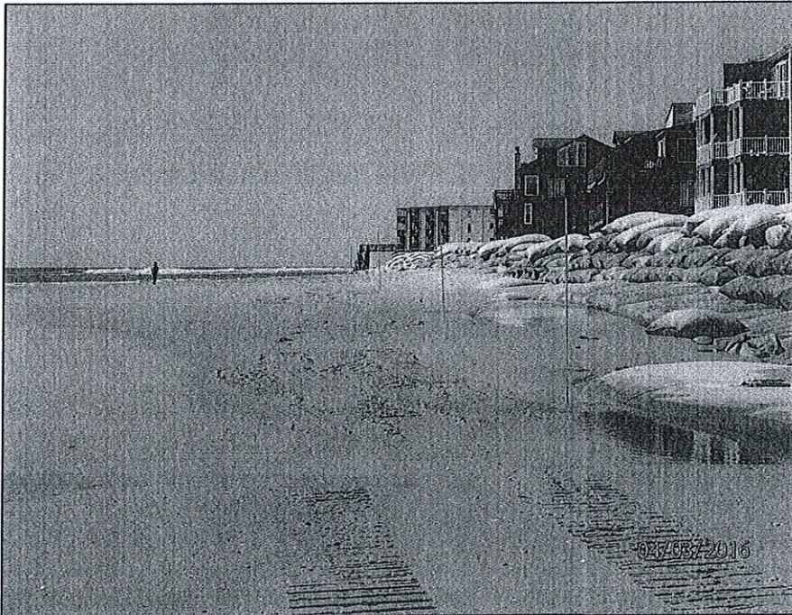
Figure 10. April 3, 2016 photo showing poles placed by the dredge contractor marking the landward location of sand to be placed during the navigation maintenance project construction.
