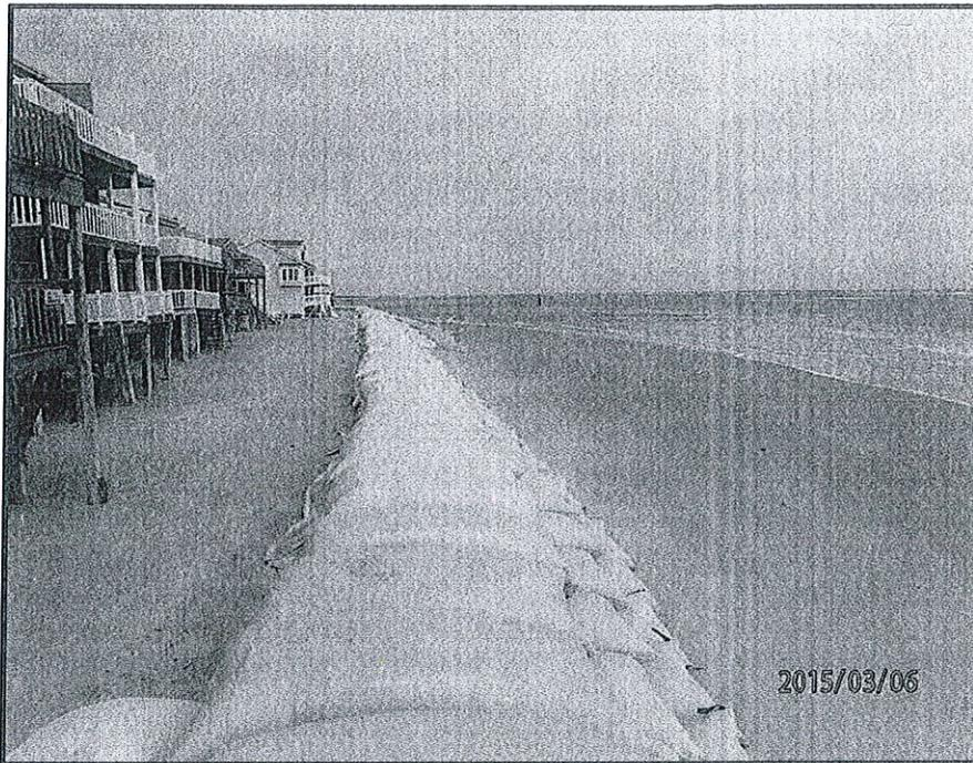
Figure 7. March 6, 2015 photo showing buried sand tube along south end of sandbag revetment.
