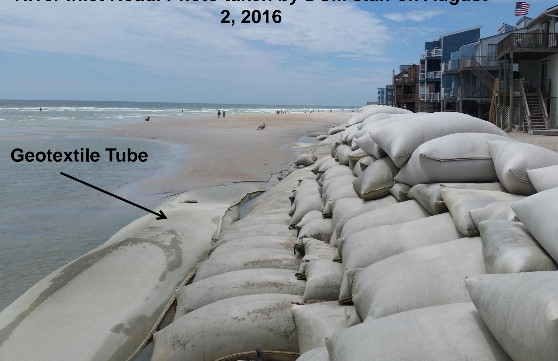
**Photo of Geotextile Tube looking north from 2368 New River Inlet Road. Photo taken by DCM staff on August 2, 2016.**
