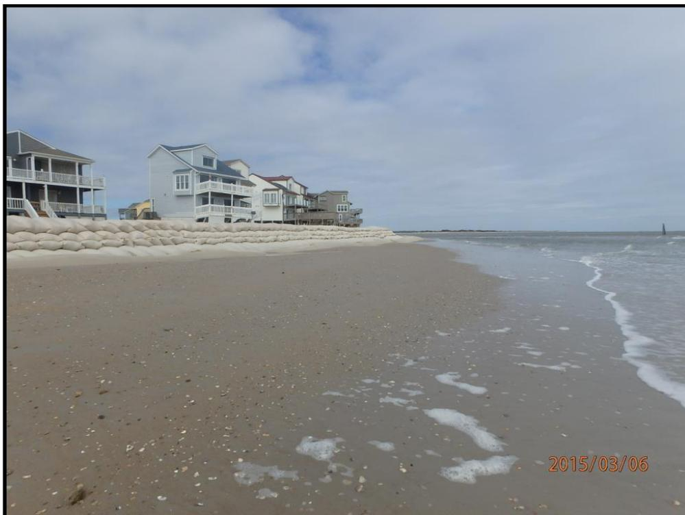
Figure 5 – March 6, 2015 photo of sandbag revetment and partially buried sand tube
