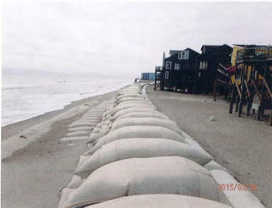
Figure 5. March 6, 2015 photo of sandbag revetment and partially buried sand tube near middle of sandbag revetment.
