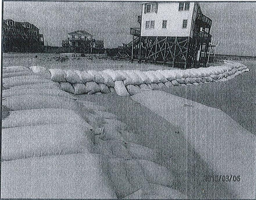
Figure 3. March 6, 2015 photo of sandbag revetment and sand tube at north end of revetment.
