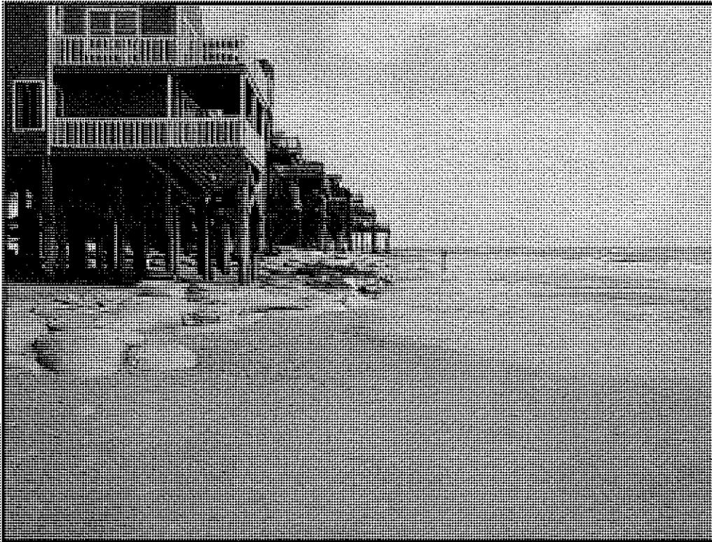
**Figure 14. Example of failed sandbag revetment on north end of North Topsail Beach.**
