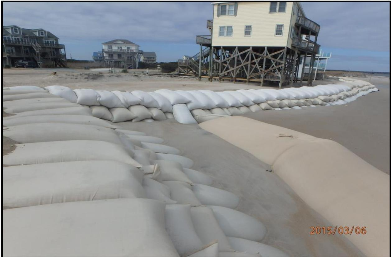
**Figure 3 – March 6, 2015 photo of sandbag revetment and sand tube at north end of revetment.**
