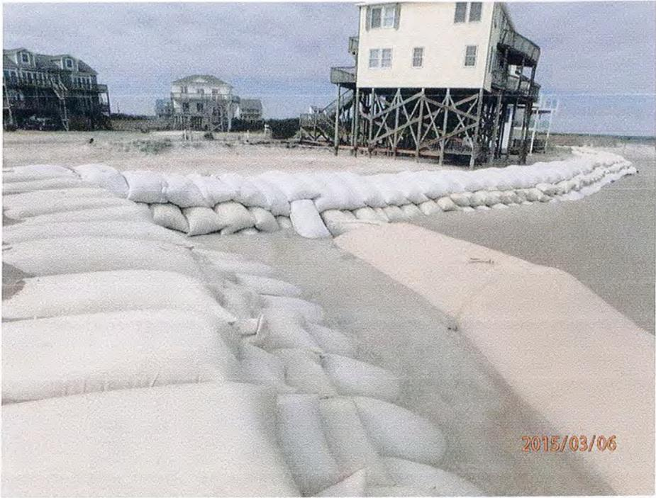
Figure 2. March 6, 2015 photo of sandbag revetment and sand tube at north end of revetment.
