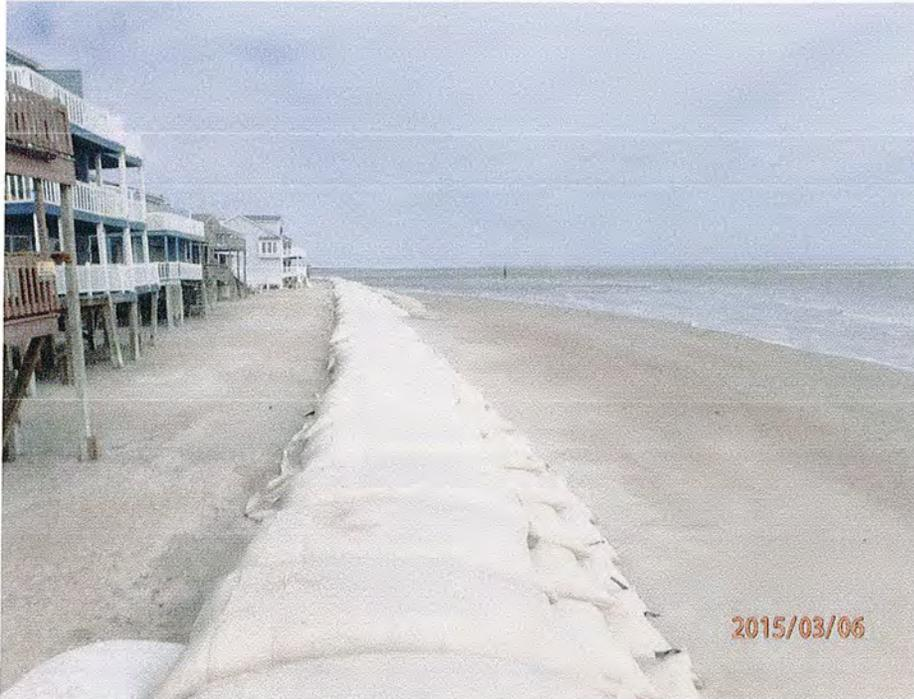
**Figure 6. March 6, 2015 photo showing buried sand tube along south end of sandbag revetment.**
