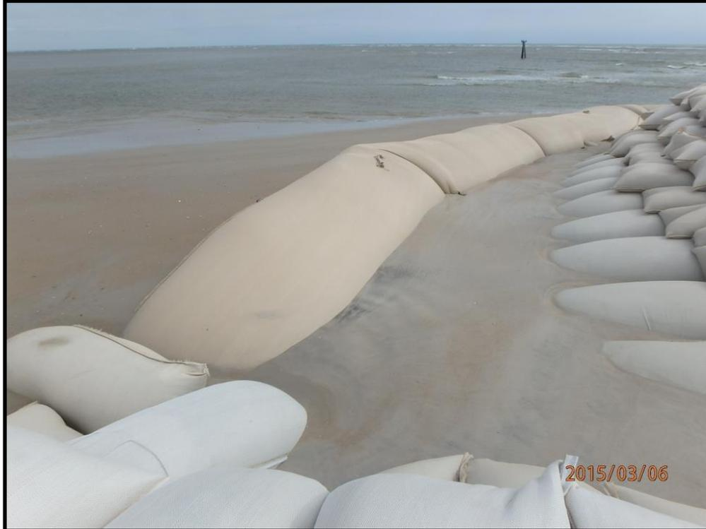
Figure 4 – March 6, 2015 photo of sandbag revetment and sand tube at north end of revetment.
