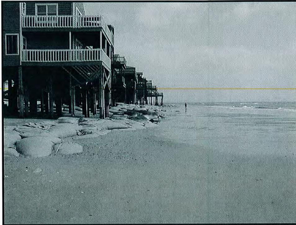
**Photo 7. Example of failed sandbag revetment on north end of North Topsail Beach. Photo taken in September 2005. All of these sandbags and structures, which were located seaward of the present row of homes north of Topsail Reef, have been removed.**
