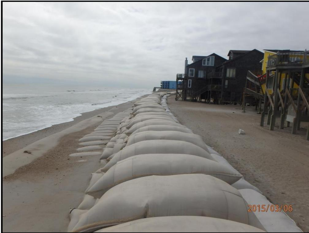
**Figure 6 – March 6, 2015 photo of sandbag revetment and partially buried sand tube near the middle of the sandbag revetment**
