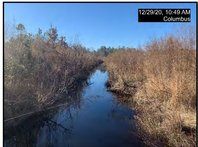
Looking upstream along Cow Branch showing channelized conditions.
