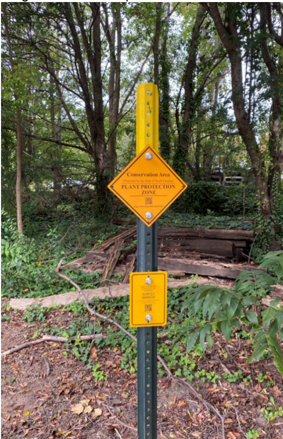
Installed witness post example.
