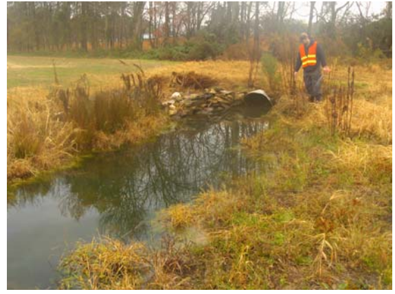
Photo Point 8. Pipe at outlet at existing Farm Crossing Lower Reach
