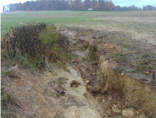
Photo Point 1. Uppermost head cut top of project- Ephemeral Channel
