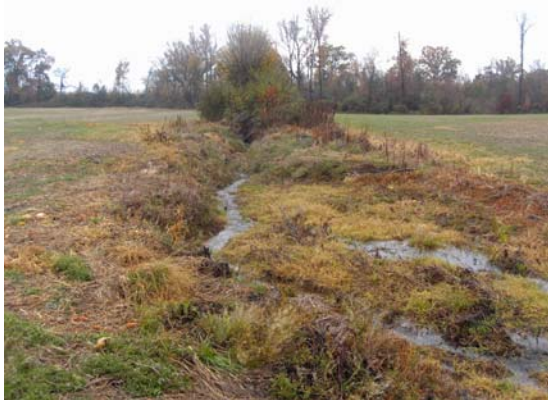
Photo Point 9. Existing channel at outlet of plunge pool at farm crossing viewing incised channel downstream
