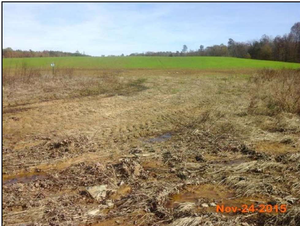
Project Reach 3 – Encroachment 45+50
