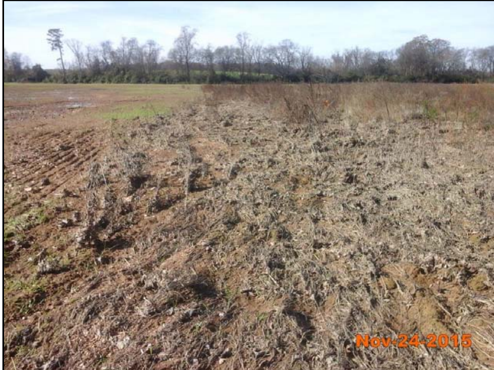
Project Reach 3 – Encroachment 47+50 Left Descending Bank
