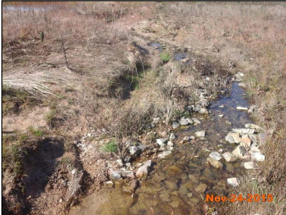
Project Reach 1 – Bank Erosion 9+50
