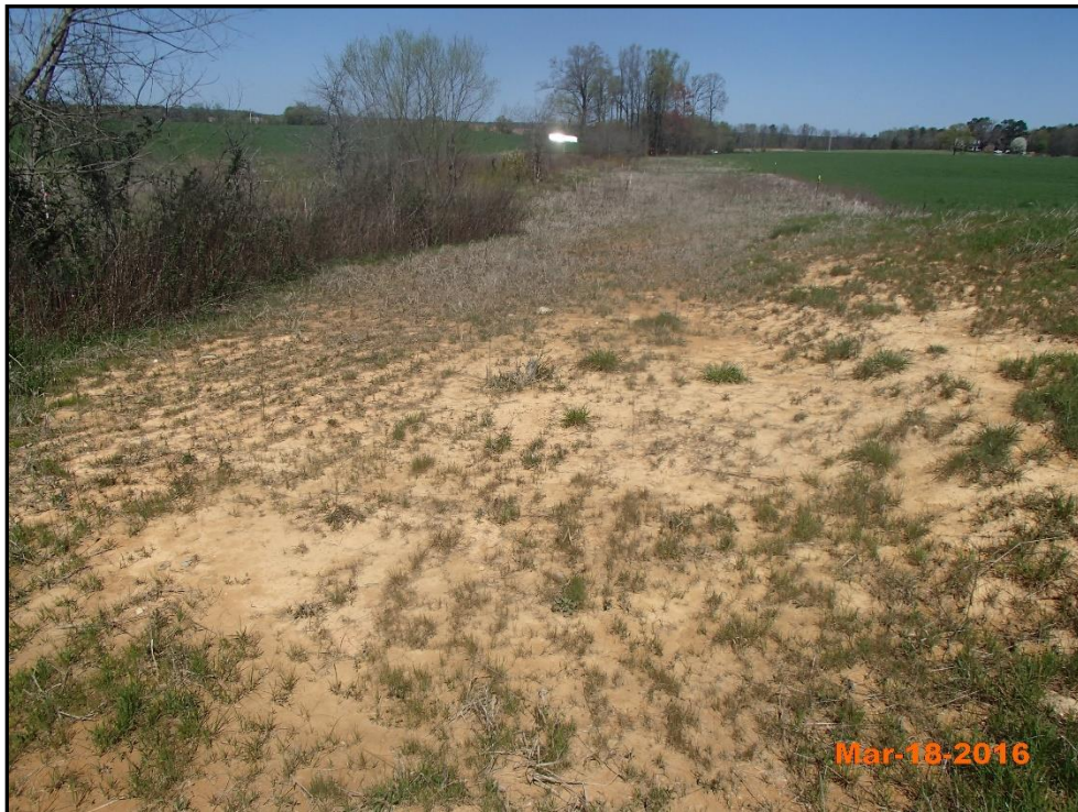
Project Reach 1 – Ditch / Bare Area 14+00 Right Descending Bank
