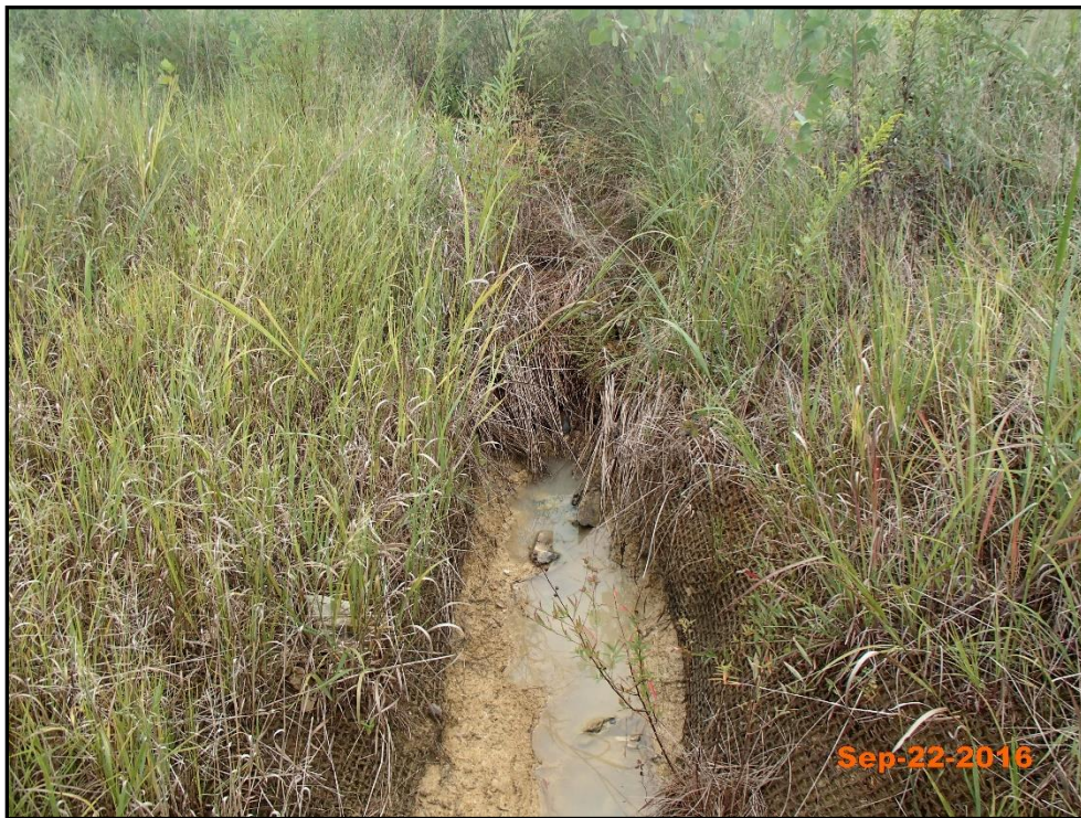
Project Reach 1 – Headcut/Degradation 9+25
