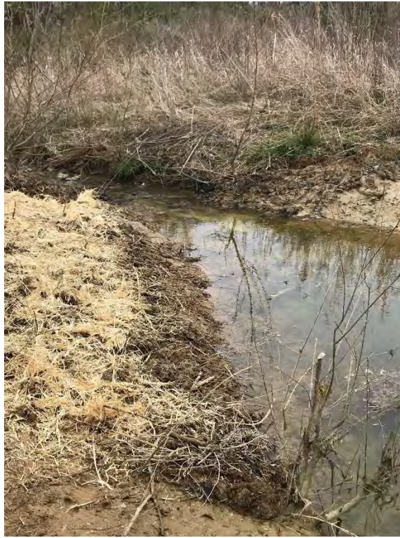
Beaver dam removal and bank stabilization near XS17. (3/27/2018)
