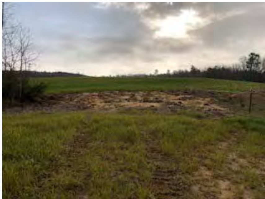
Crossing repair near VP5. (3/27/2018)
