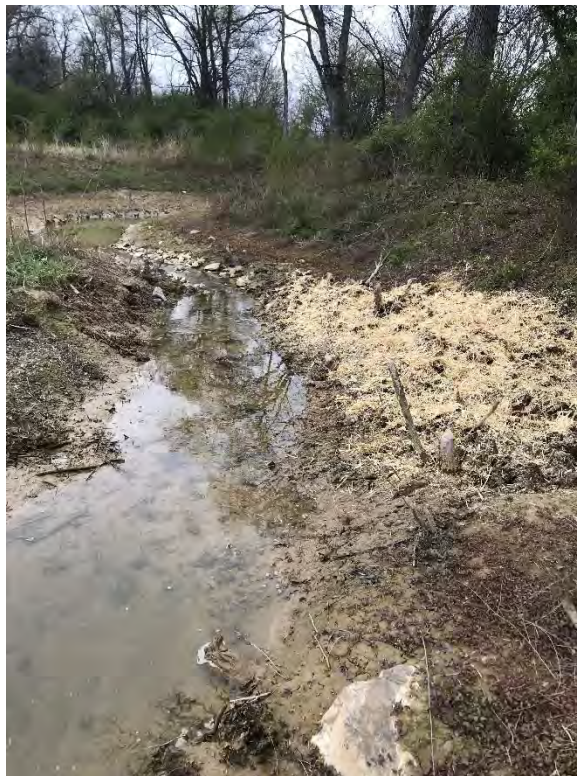
Beaver dam removal and bank stabilization downstream of XS18. (3/27/2018)
