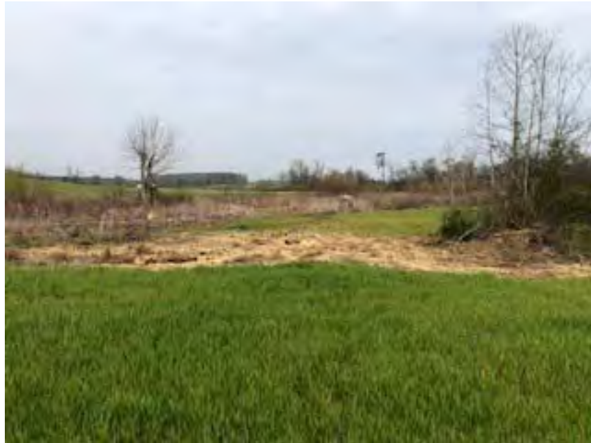
Crossing repair near VP5. (3/27/2018)
