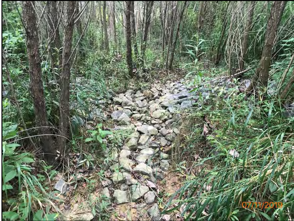
Reach 1 – Permanent Photo Station 1 Top of Project – Looking Downstream
