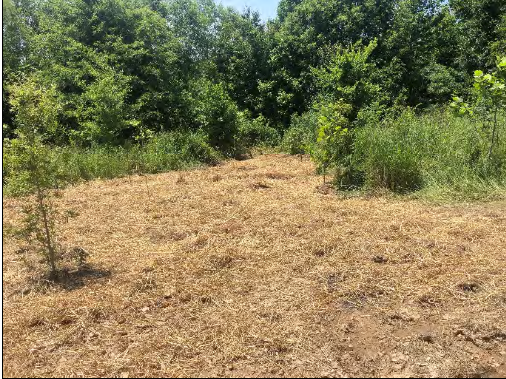
Headcut repair with seeding and coir logs
