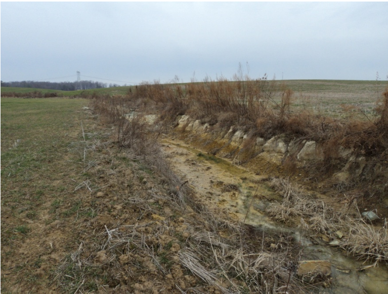
Photo 3. Wicker Branch - Bank erosion
