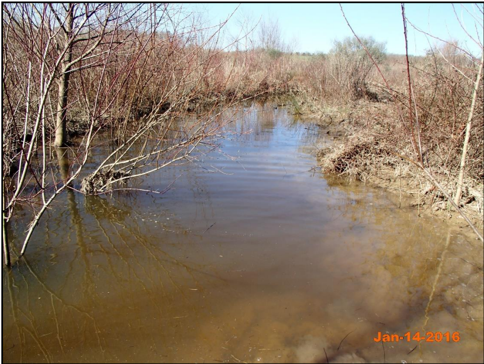
Project Reach 2 – Beaver Dam (removed) 11+00 Looking Upstream
