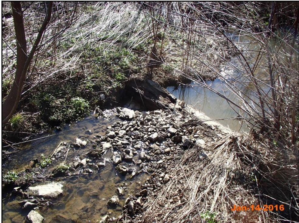
Project Reach 5 – Stressed Structure 13+25 Looking Downstream
