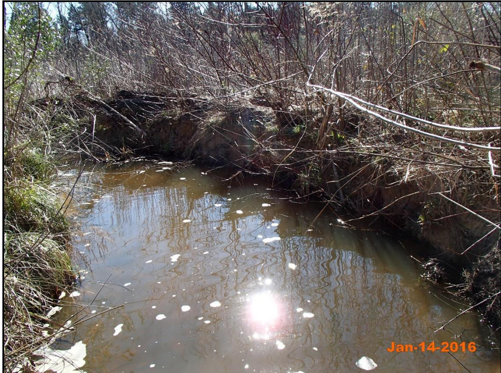
Project Reach 2 – Bank Erosion 19+50 Right Descending Bank
