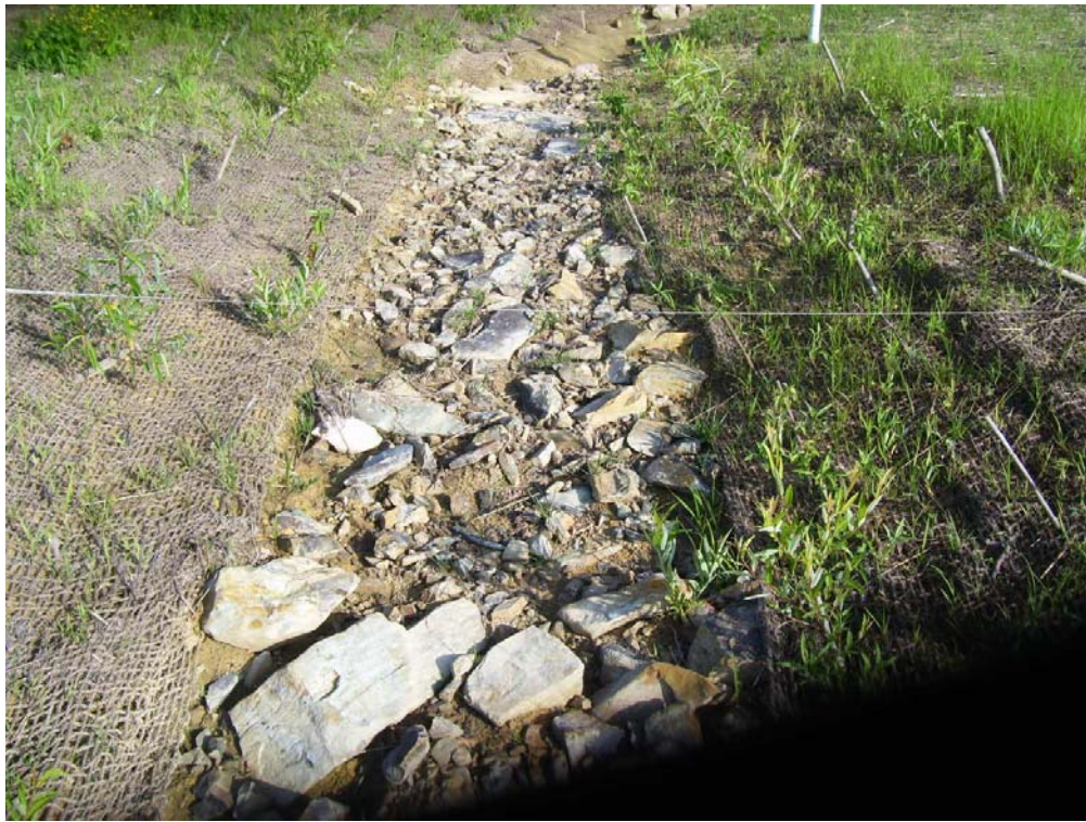
RXS2: Looking Upstream (May 29, 2008)
