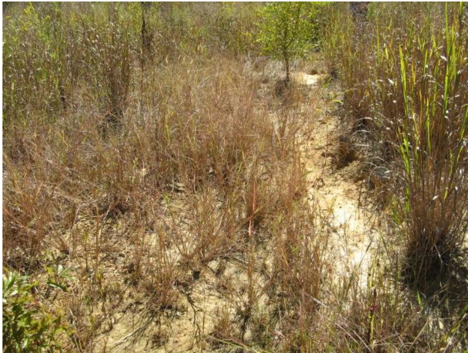
Problem Area Photo 4
