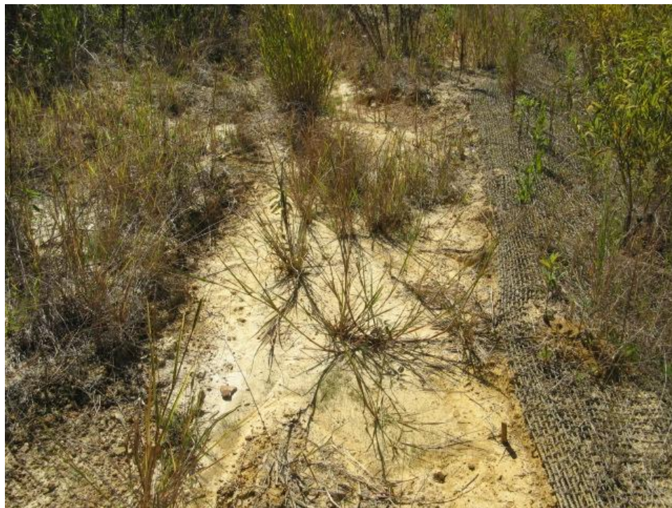
Problem Area Photo 6
