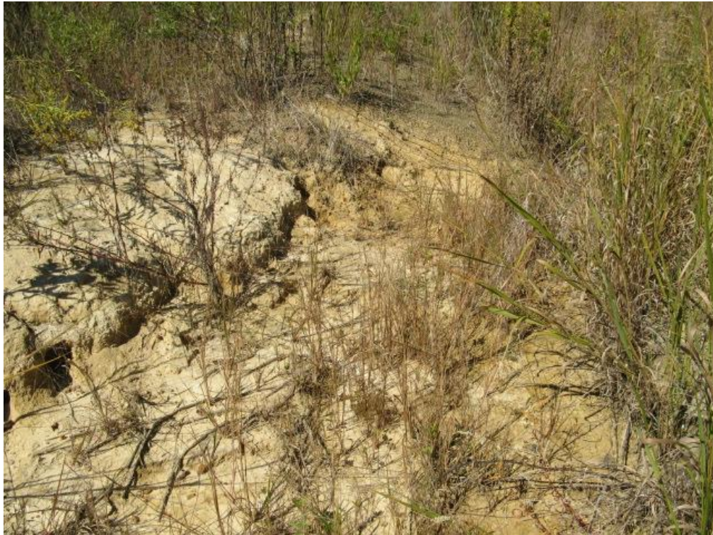
Problem Area Photo 9
