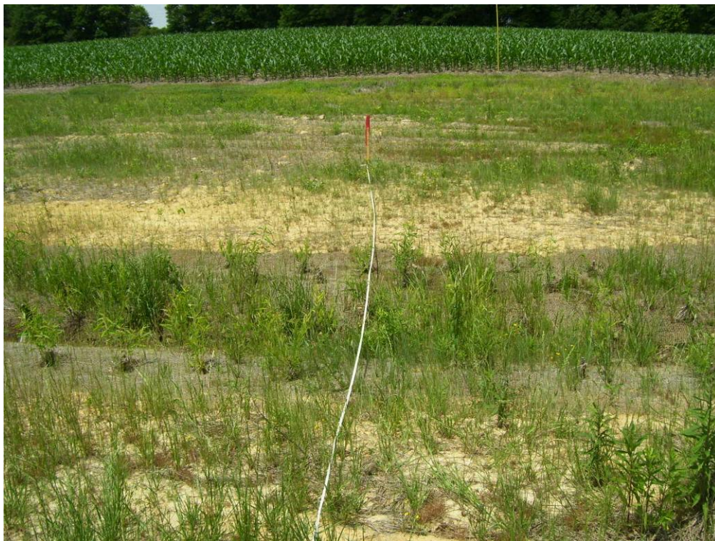
R1 RXS1: Looking at Left Bank (May 29, 2008)
